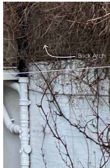
2B. Original ground floor brick arch.
