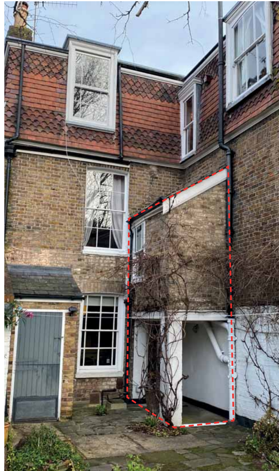
3. Rear Elevation. WC Extension removed
