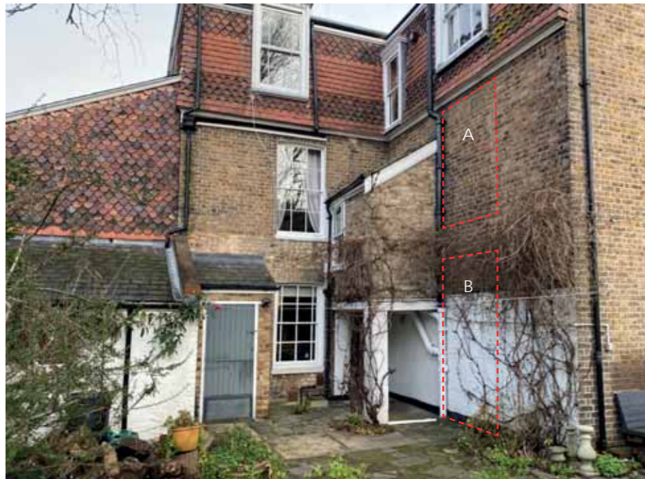
2. Rear Elevation. Brick Lintels indicate location of original windows.
