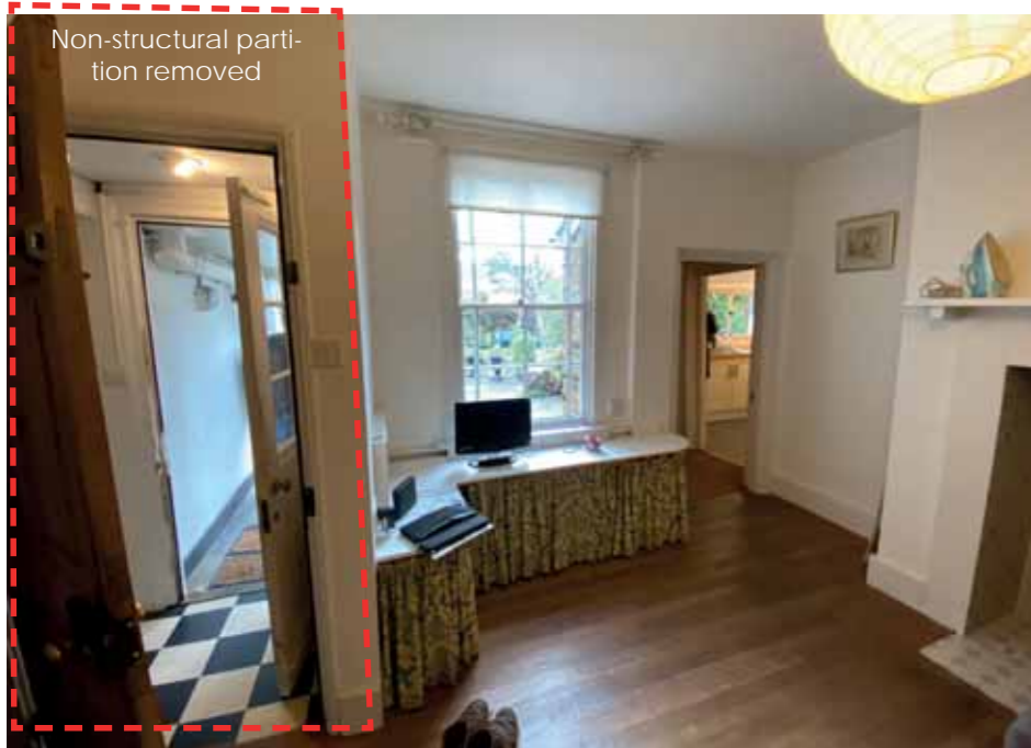
4. Internal Partition removed
