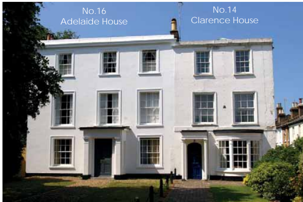
Adelaide House, 16 Park Road/ (Left)
