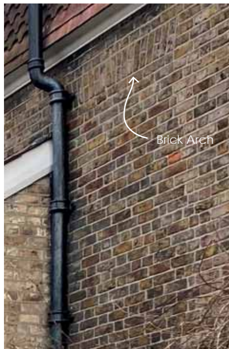
2A. Original 1st floor brick arch.
