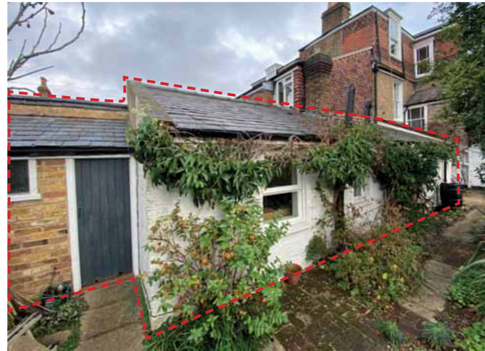
1. Existing Rear Building
