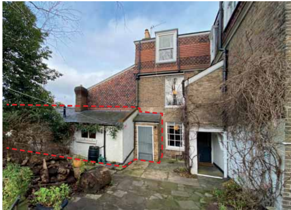
1. Existing Rear Building
