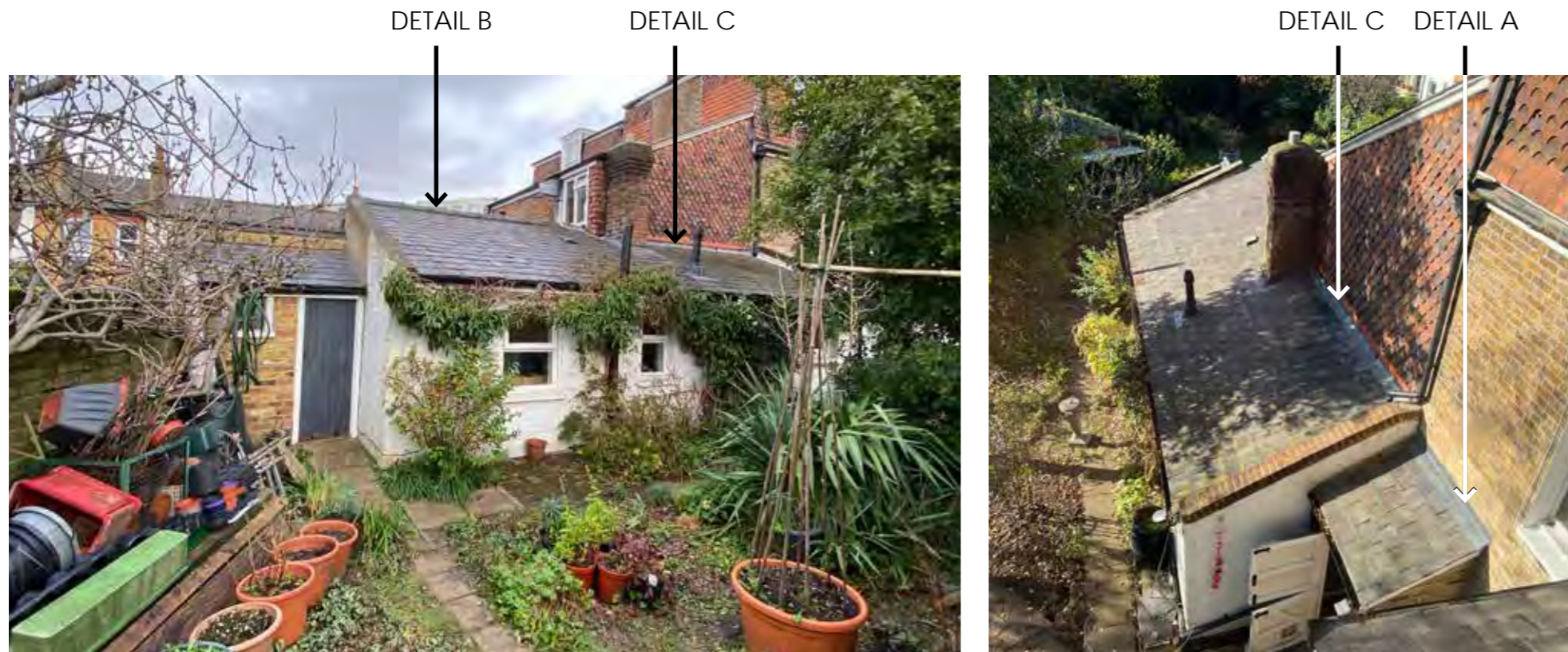
Photos of Existing Rear extension
