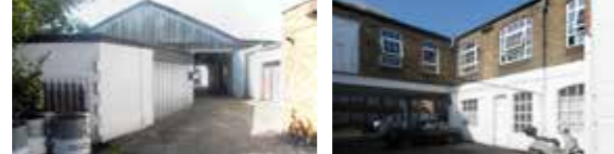
Existing site photos
