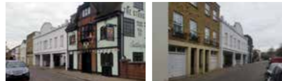
Existing site photos
