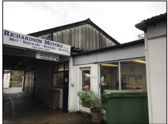
Image 6: Buildings within the site boundary.
