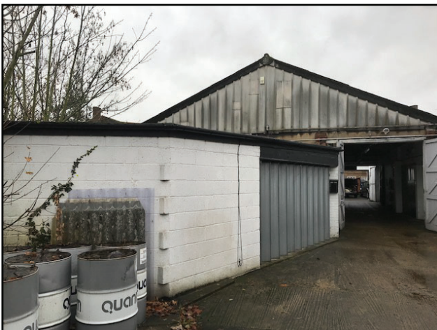
Image 7: Buildings within the site boundary.
