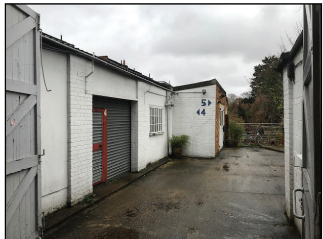
Image 4: An area of buildings and hardstanding present on site.
