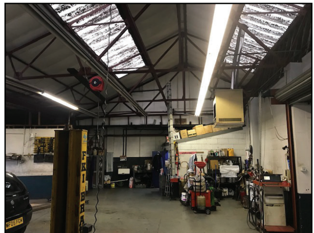
Image 8: Internal of a building within the site boundary.
