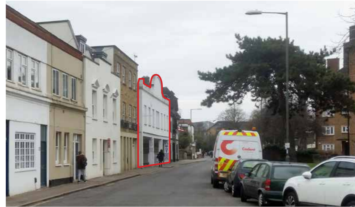
View from North-West along Priests Bridge As Existing
