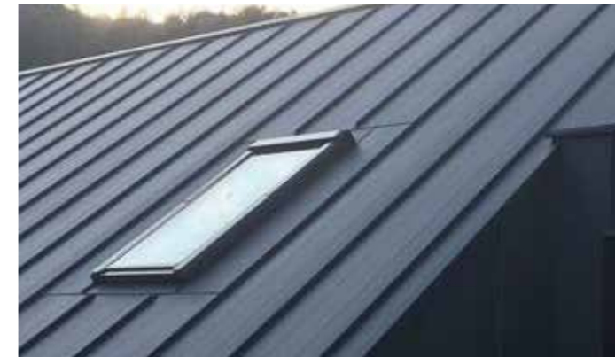
01 Profiled coated steel roofing
