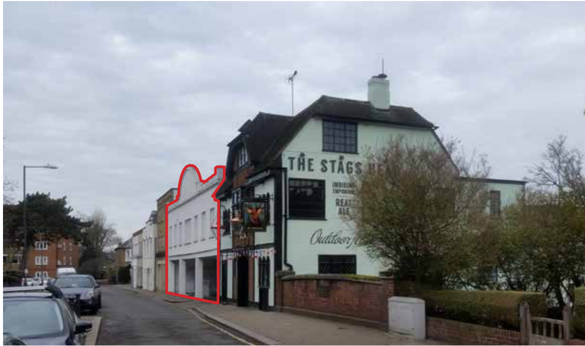
View from South-East along Priests Bridge As Existing
