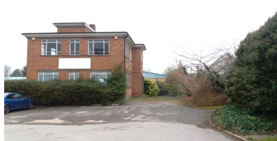
5. Holly House in the centre of the site, southern elevation
