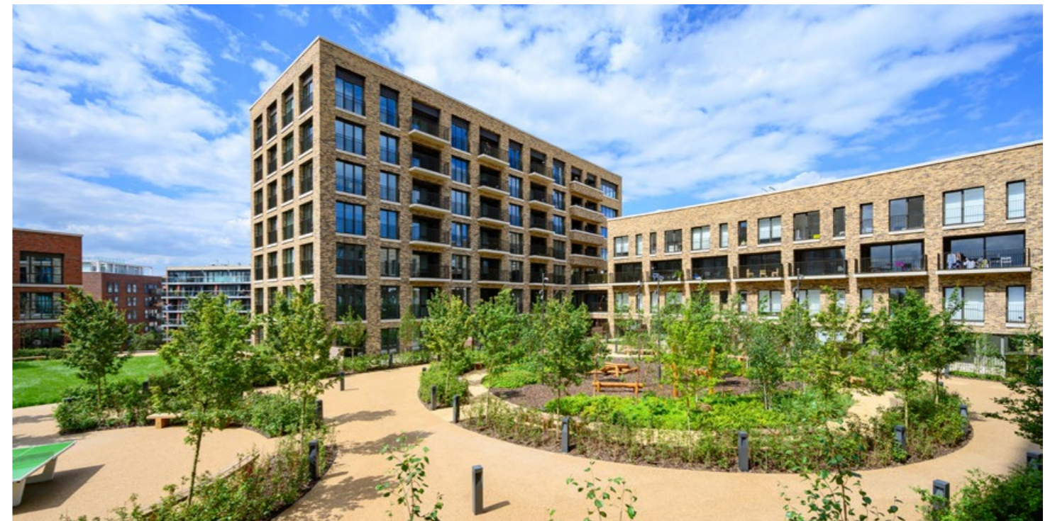
The Water Yards, Canada Water, Southwark - mixed-use scheme by Notting Hill Genesis
