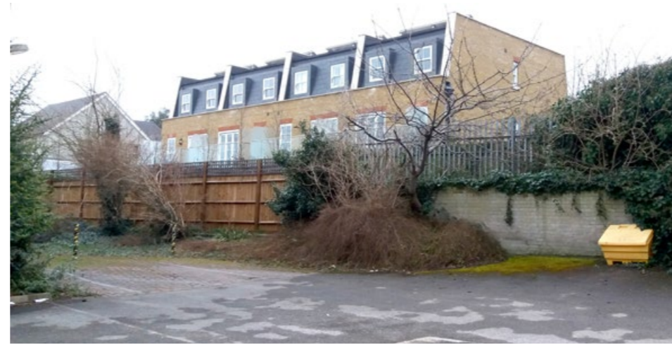
2. Rear gardens of Penny Farthing Mews seen from the site
