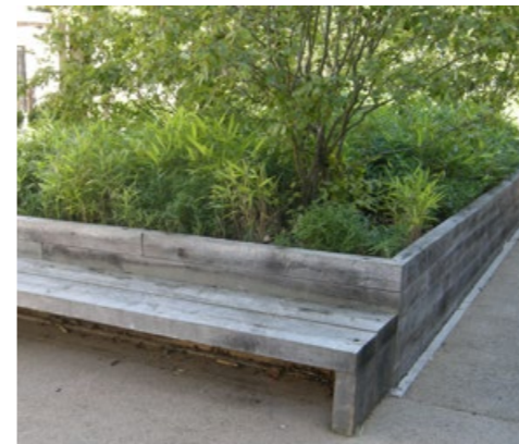
Raised podium planters
