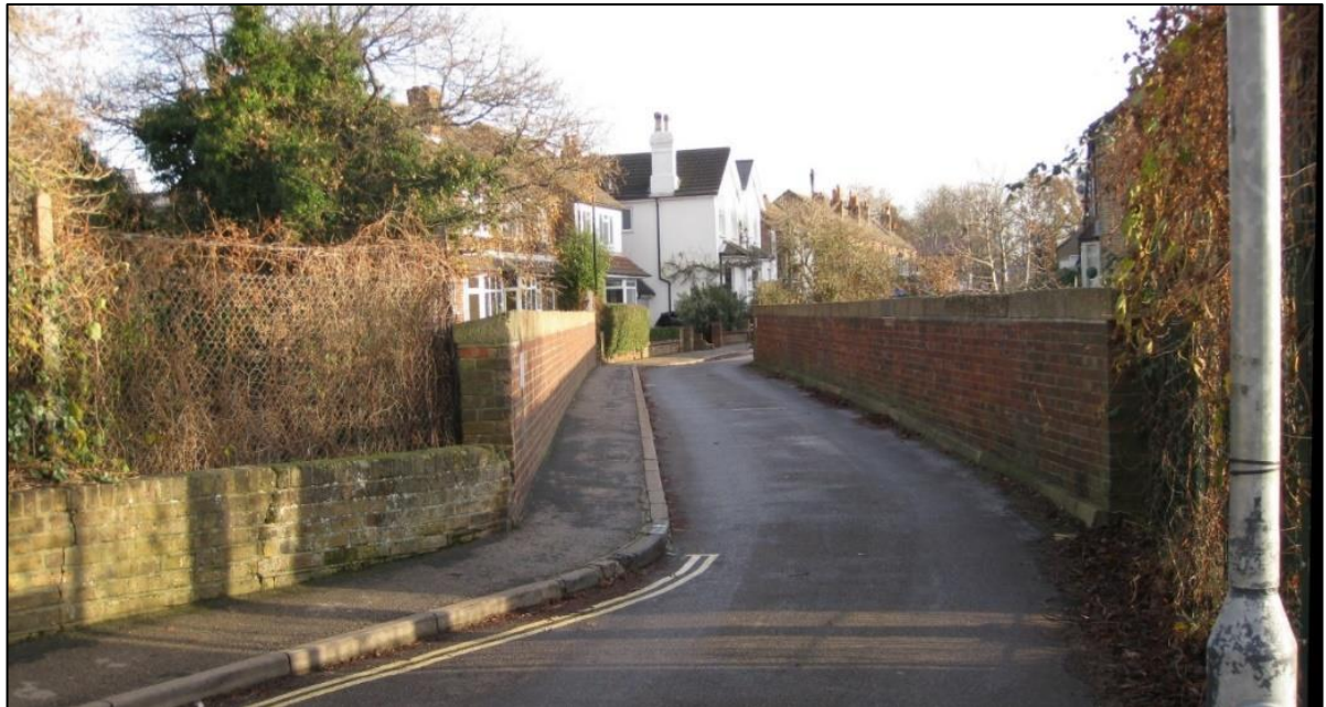
Figure 2.2 - Railway bridge between Holly Road and School Road Avenue
