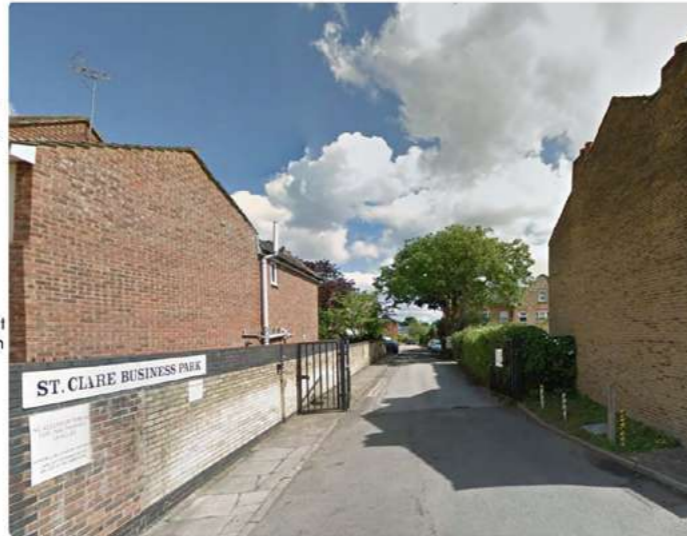
Photo of the existing site entrance from Holly Road
