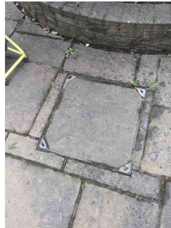
MH.15 POST SURVEY
