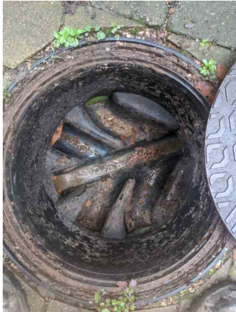
_50-56 SHEEN ROAD_RICHMOND_27_038.jpg, 00:00:00, 0.00 m Start node, manhole, reference: MH.11
