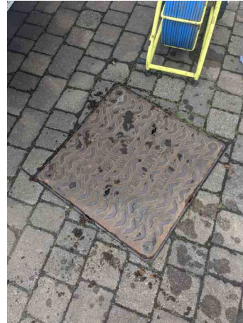
MH.24 POST SURVEY
