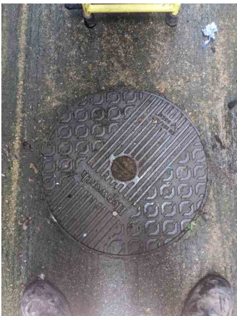
MH.12 POST SURVEY
