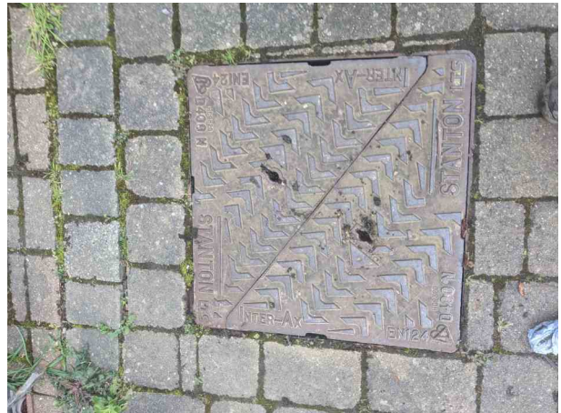
MH.23 POST SURVEY
