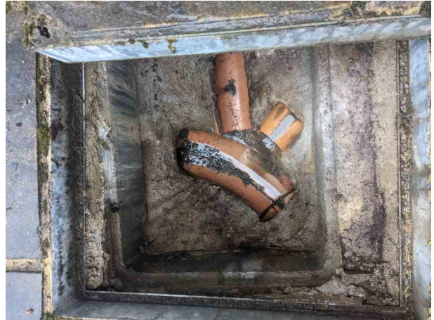
_50-56 SHEEN ROAD_RICHMOND_23_032.jpg, 00:00:57, 8.53 m Finish node, manhole, reference: MH.10
