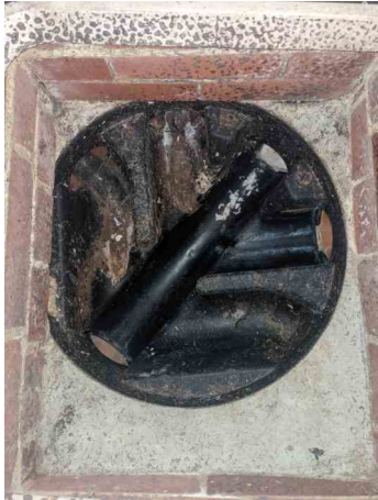
_50-56 SHEEN ROAD_RICHMOND_9_013.jpg, 00:00:00, 0.00 m Start node, manhole, reference: MH.3
