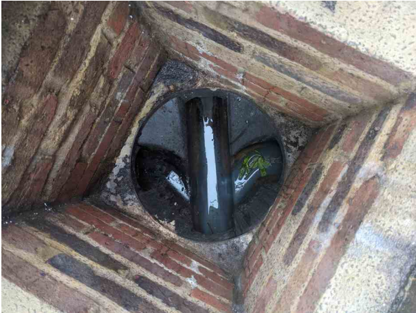
_50-56 SHEEN ROAD_RICHMOND_23_031.jpg, 00:00:00, 0.00 m Start node, manhole, reference: MH.2
