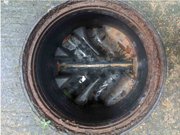
_50-56 SHEEN ROAD_RICHMOND_28_040.jpg, 00:00:00, 0.00 m Start node, manhole, reference: MH.12
