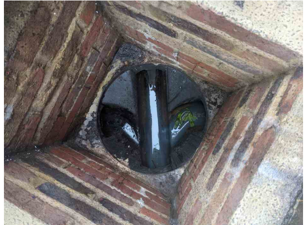
_50-56 SHEEN ROAD_RICHMOND_18_027.jpg, 00:00:30, 6.77 m Finish node, manhole, reference: MH.2
