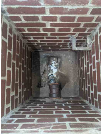
_50-56 SHEEN ROAD_RICHMOND_15_022.jpg, 00:00:00, 0.00 m Start node, manhole, reference: MH.5
