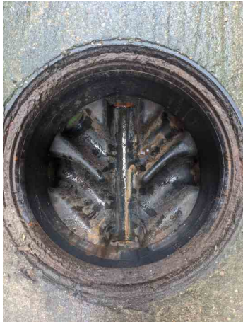
_50-56 SHEEN ROAD_RICHMOND_29_042.jpg, 00:00:00, 0.00 m Start node, manhole, reference: MH.13
