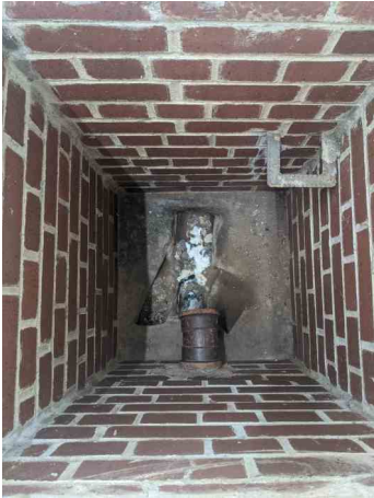
_50-56 SHEEN ROAD_RICHMOND_16_023.jpg, 00:00:00, 0.00 m Start node, manhole, reference: MH.5
