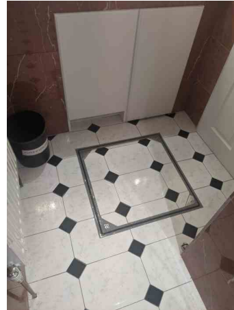
MH.1 POST SURVEY
