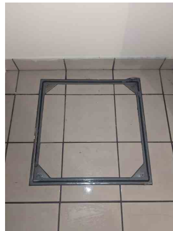
MH.3 POST SURVEY
