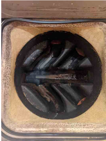
_50-56 SHEEN ROAD_RICHMOND_2_003.jpg, 00:00:00, 0.00 m Start node, manhole, reference: MH.1
