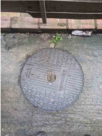
MH.13 POST SURVEY
