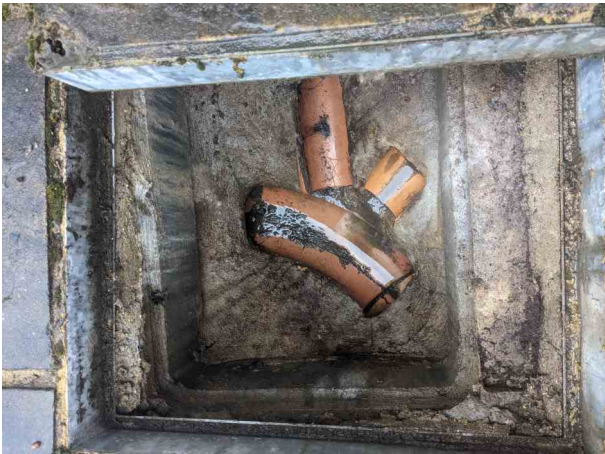
_50-56 SHEEN ROAD_RICHMOND_25_035.jpg, 00:00:00, 0.00 m Start node, manhole, reference: MH.10
