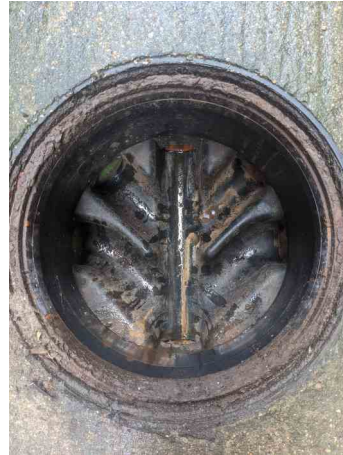
_50-56 SHEEN ROAD_RICHMOND_28_041.jpg, 00:00:07, 1.39 m Finish node, manhole, reference: MH.13
