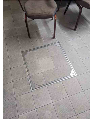
MH.4 POST SURVEY
