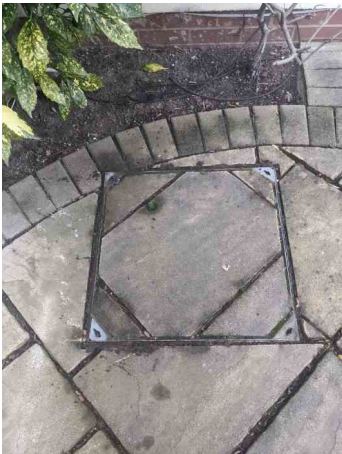
MH.9 POST SURVEY
