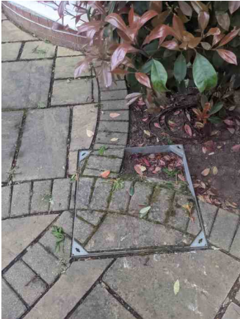
MH.7 POST SURVEY
