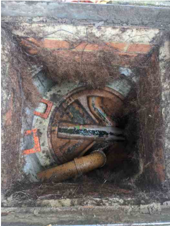
_50-56 SHEEN ROAD_RICHMOND_18_026.jpg, 00:00:00, 0.00 m Start node, manhole, reference: MH.7
