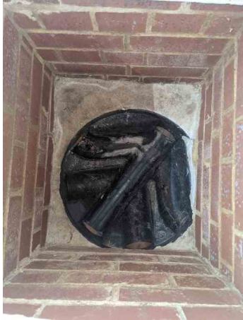
_50-56 SHEEN ROAD_RICHMOND_13_020.jpg, 00:00:00, 0.00 m Start node, manhole, reference: MH.4
