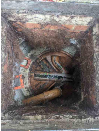
_50-56 SHEEN ROAD_RICHMOND_21_030.jpg, 00:00:00, 0.00 m Start node, manhole, reference: MH.7
