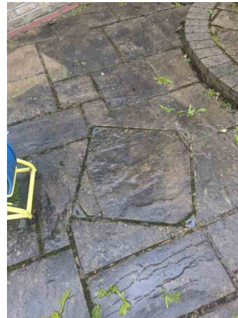
MH.2 POST SURVEY
