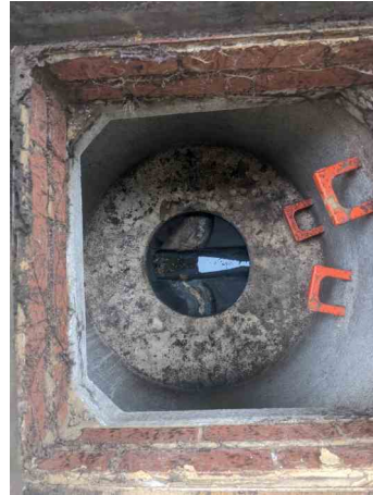
_50-56 SHEEN ROAD_RICHMOND_21_087.jpg, 00:00:14, 2.71 m Finish node, manhole, reference: MH.8
