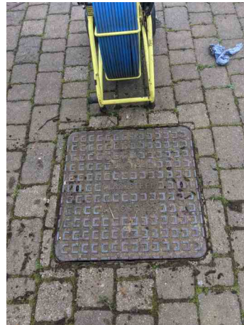
MH.21 POST SURVEY
