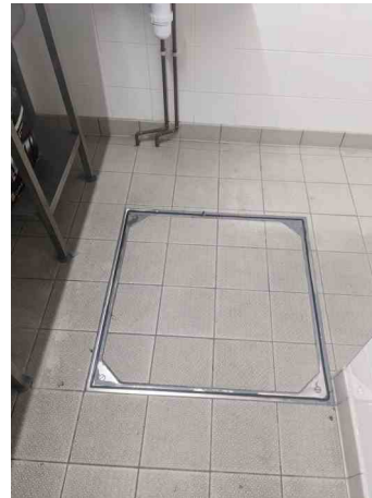
MH.5 POST SURVEY
