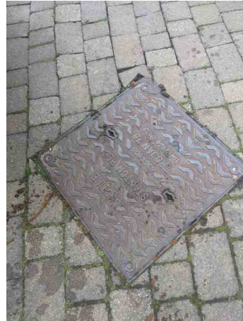
MH.20 POST SURVEY
