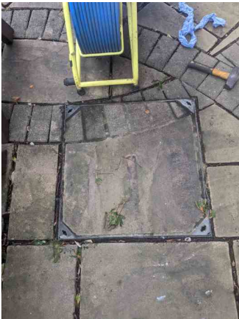
MH.8 POST SURVEY
