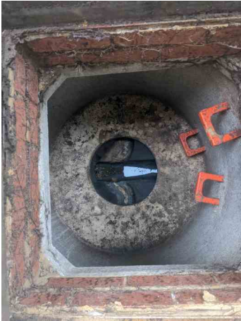
_50-56 SHEEN ROAD_RICHMOND_22_086.jpg, 00:00:00, 0.00 m Start node, manhole, reference: MH.8
