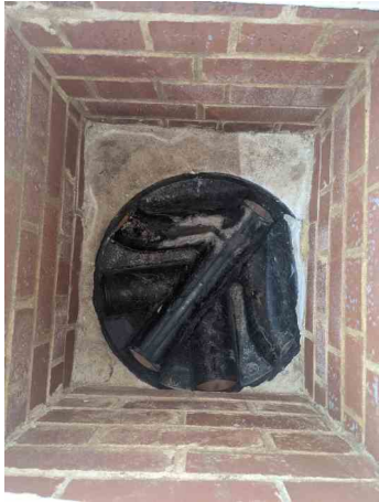
_50-56 SHEEN ROAD_RICHMOND_11_016.jpg, 00:00:00, 0.00 m Start node, manhole, reference: MH.4
