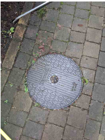
MH.11 POST SURVEY
