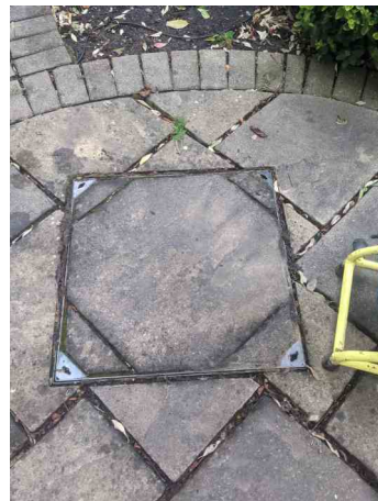
MH.19 POST SURVEY
