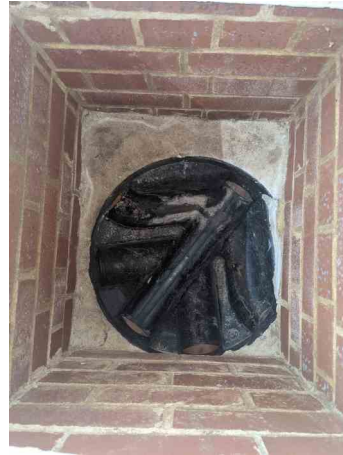
_50-56 SHEEN ROAD_RICHMOND_10_015.jpg, 00:00:20, 4.79 m Finish node, manhole, reference: MH.4
