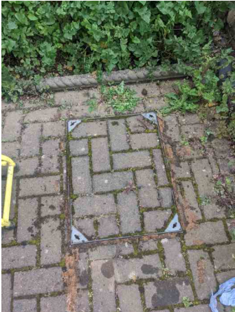
MH.27 POST SURVEY
