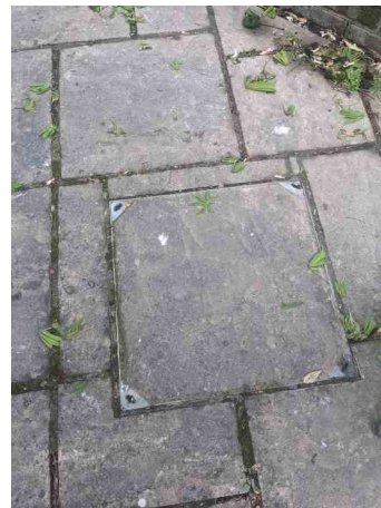
MH.16 POST SURVEY
