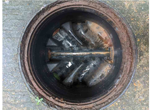
_50-56 SHEEN ROAD_RICHMOND_27_039.jpg, 00:00:18, 4.90 m Finish node, manhole, reference: MH.12
