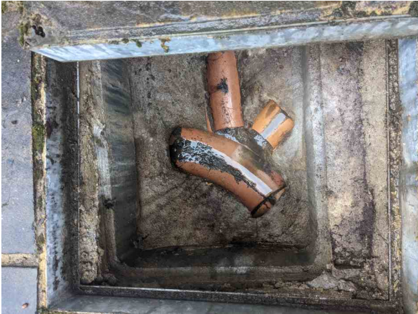
_50-56 SHEEN ROAD_RICHMOND_26_037.jpg, 00:00:00, 0.00 m Start node, manhole, reference: MH.10
