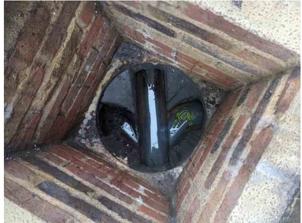
_50-56 SHEEN ROAD_RICHMOND_5_009.jpg, 00:01:17, 14.68 m Finish node, manhole, reference: MH.2
