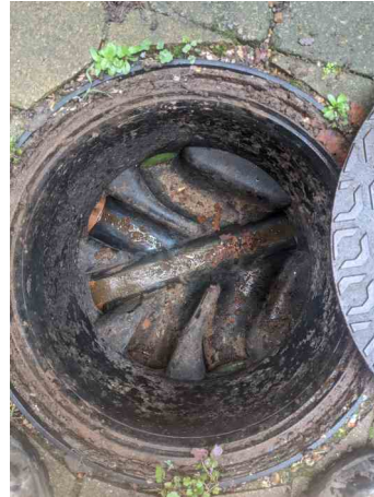
_50-56 SHEEN ROAD_RICHMOND_24_034.jpg, 00:00:48, 12.70 m Finish node, manhole, reference: MH.11
