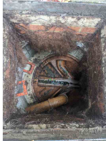
_50-56 SHEEN ROAD_RICHMOND_17_025.jpg, 00:00:36, 7.87 m Finish node, manhole, reference: MH.7
