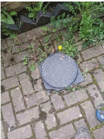
MH.26 POST SURVEY
