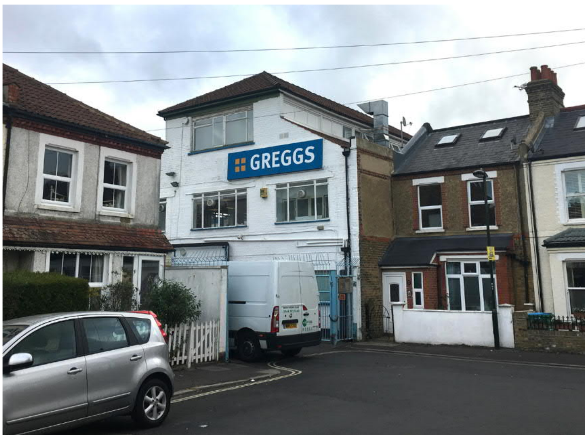
Figure 3-3: Existing access on Crane Road/Gould Road
