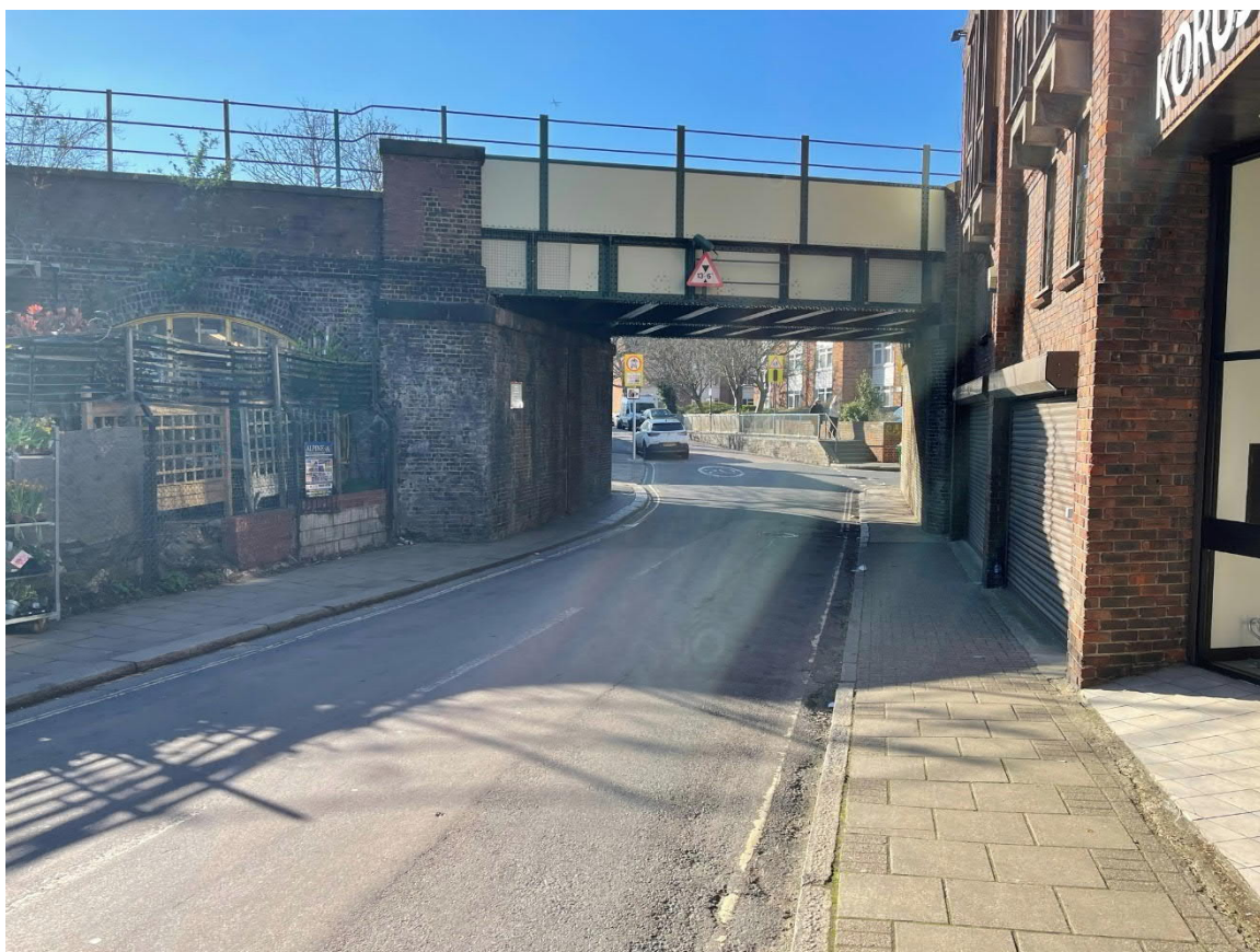
Figure 4-8: Key journey 1 – the worst point on Colne Road
