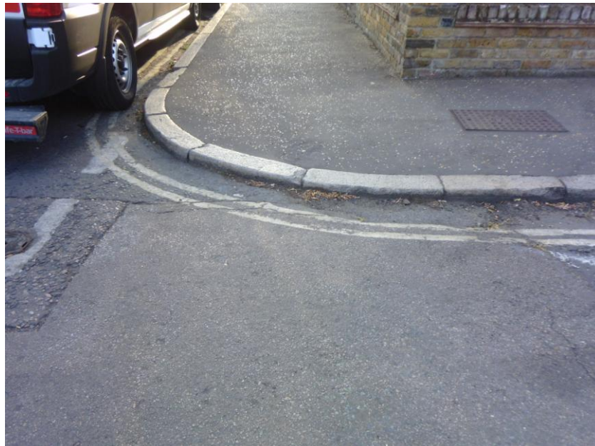
Eastern side of the May Road junction with Gould Road
