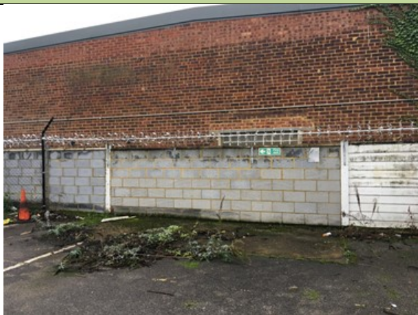
Photo 9: Examples of walls
