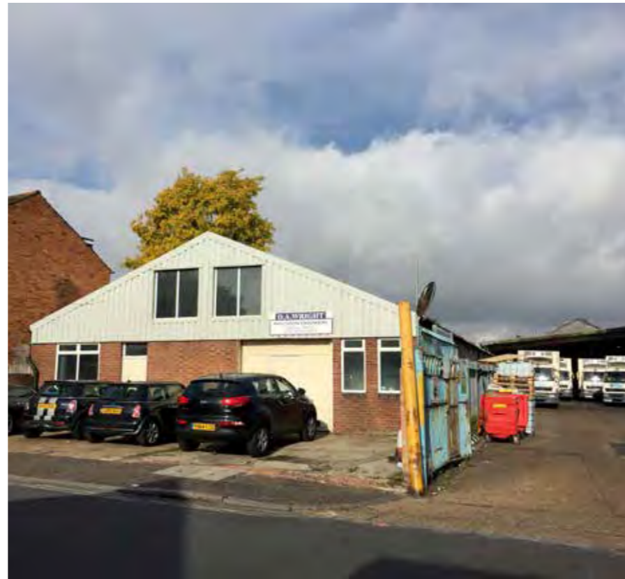
7. View looking north west of the commercial unit within site adjacent to Edwin Road entrance
