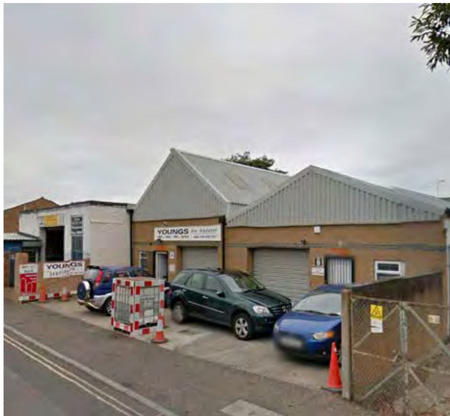
6. View looking east of commercial units opposite Edwin Road entrance
