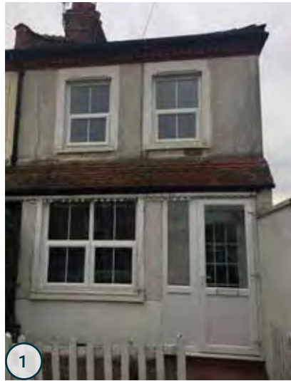
Existing house - No. 1 Gould Road
