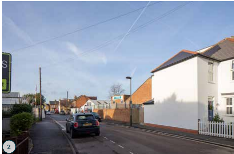
2 Southern pavement of the junction between Warwick Road and Edwin Road, looking northwest
