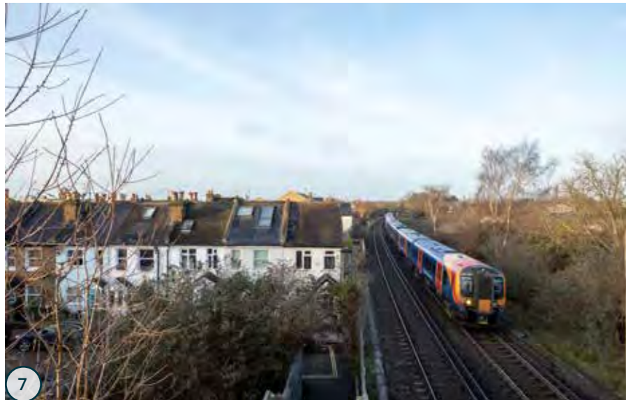
7 Footbridge crossing the railway, looking southwest
