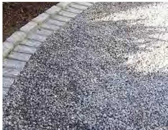
Example of gravel filled grasscrete
