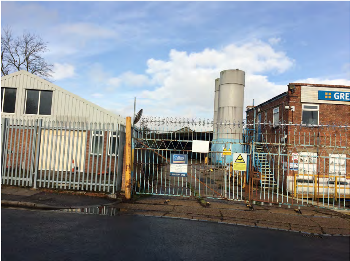
Plate 1: Edwin Road entrance viewed North with flour silo's mid distance.
