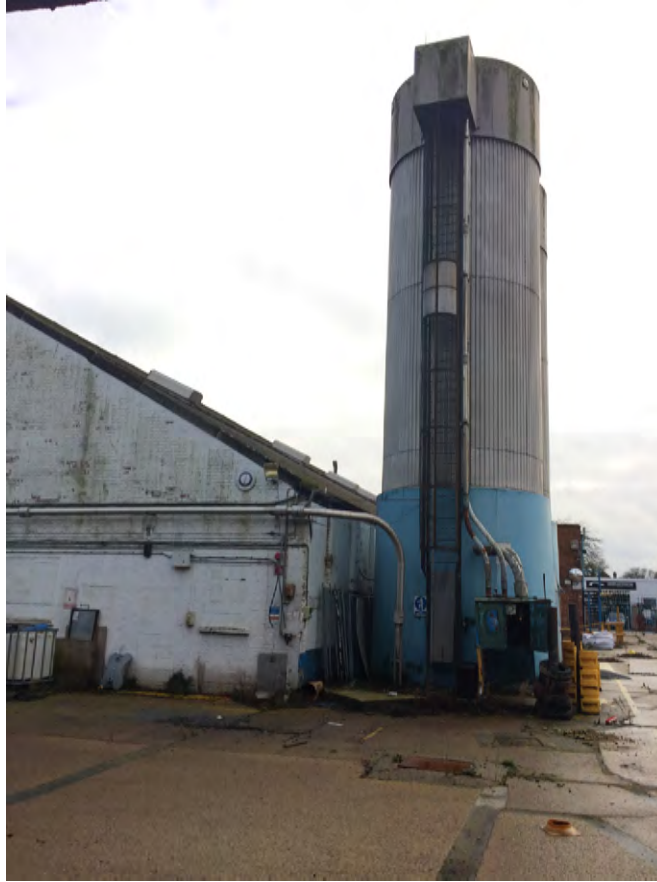
Plate 13: Northern flour Silo viewed from the North.
