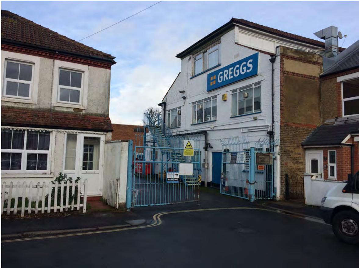
Plate 3: Gould Road administration block viewed from south-west.
