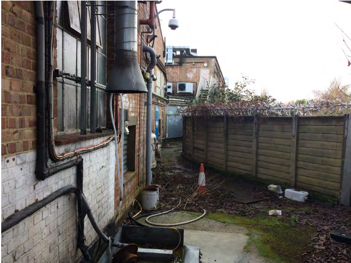
Plate 9: River frontage viewed from the east to west. River crane immediately north of the fence line.
