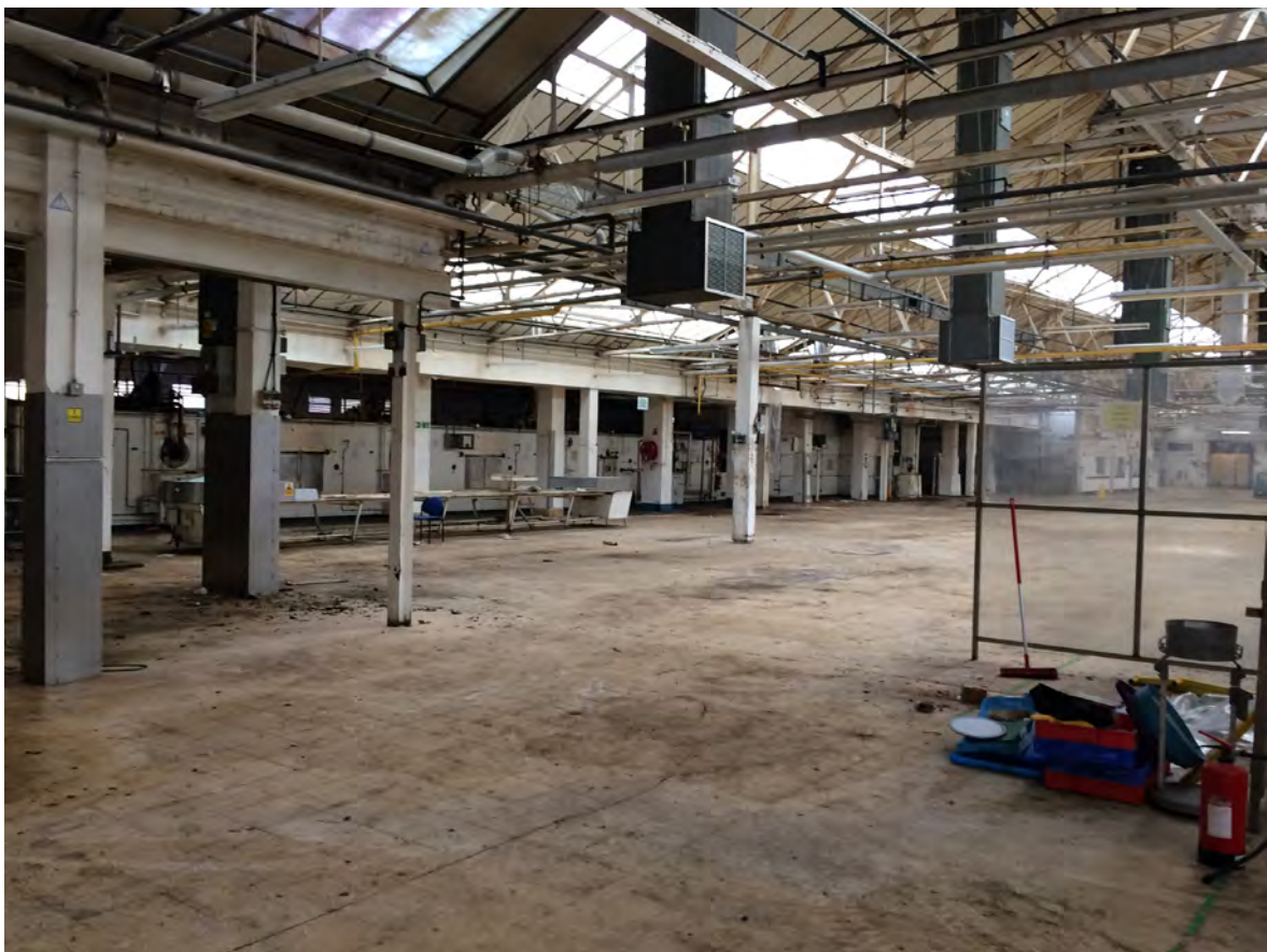
Plate 8: Oven rank along eastern edge of the site viewed from the north-west.
