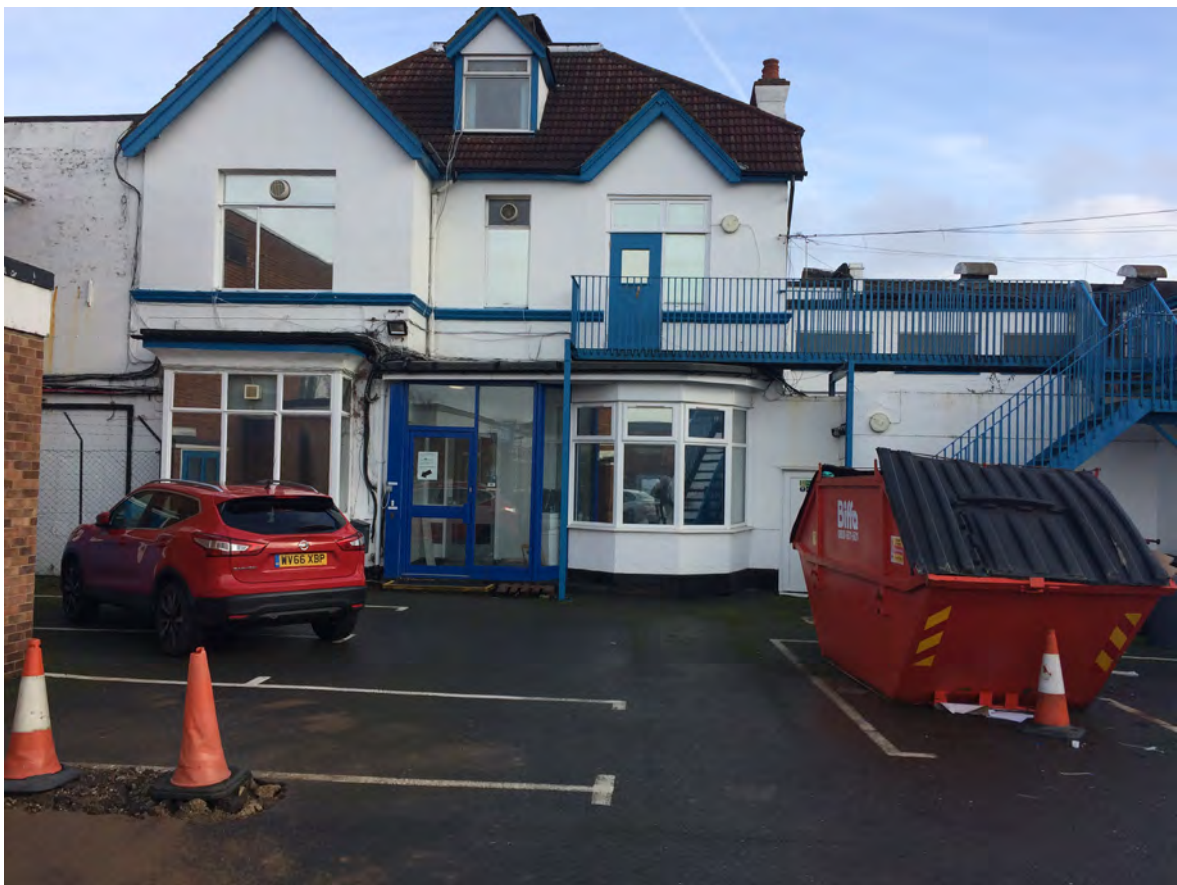
Plate 4: Gould Road northern range of administration buildings viewed from the south. Canalized River Crane immediately behind.
