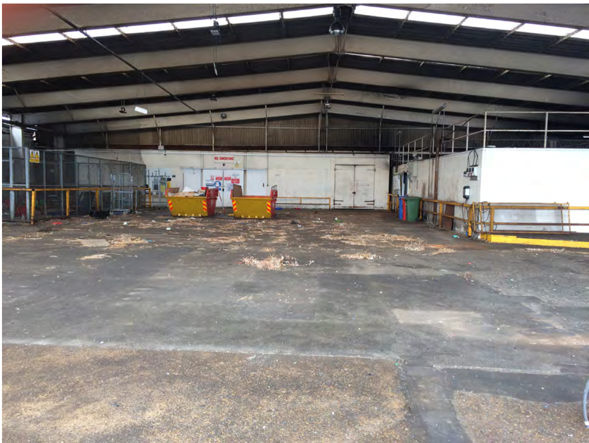
Plate 12: Edwin Road loading bays viewed from the South.
