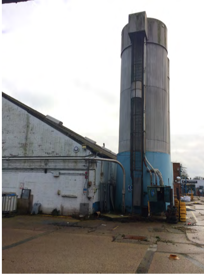
Plate 13: Northern flour Silo viewed from the North.
