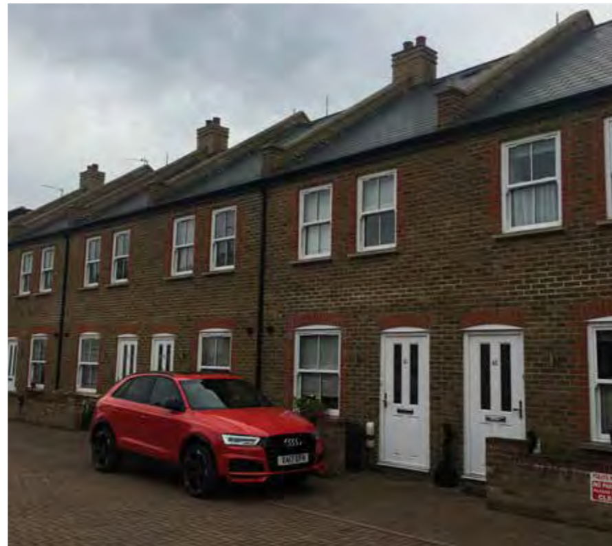
Photos of Norcutt House and terraced houses
