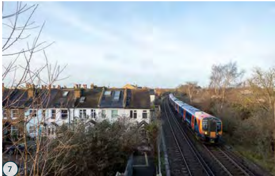
7 Footbridge crossing the railway, looking southwest
