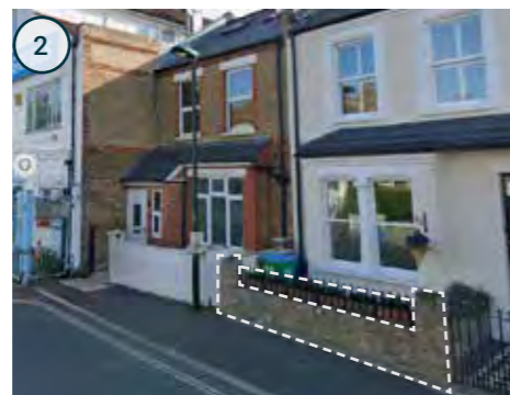
Metal fence on brick piers
