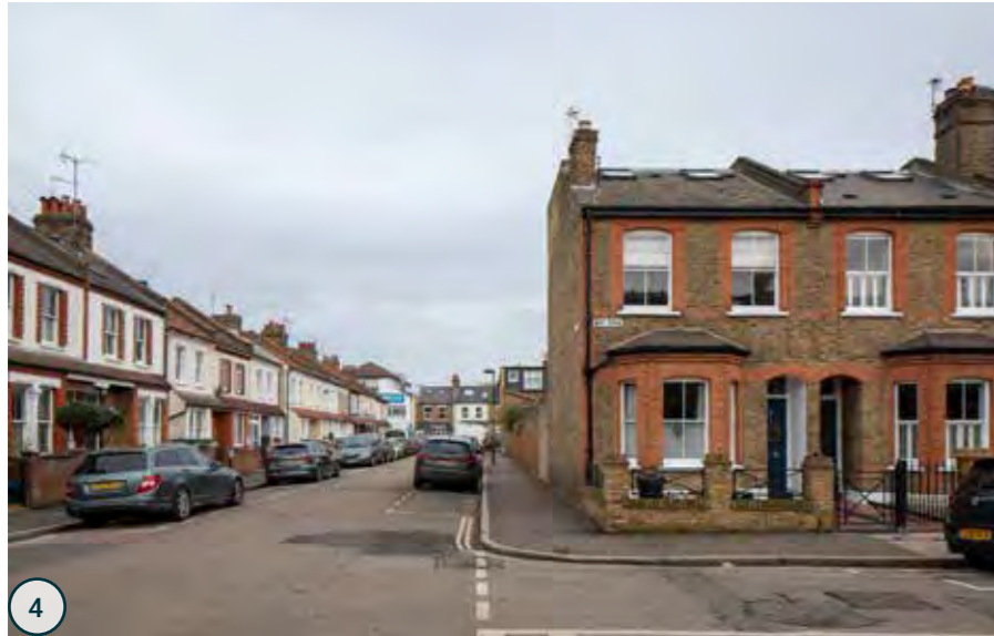
4 South western pavement of the junction between Gould Road and May Road, looking east
