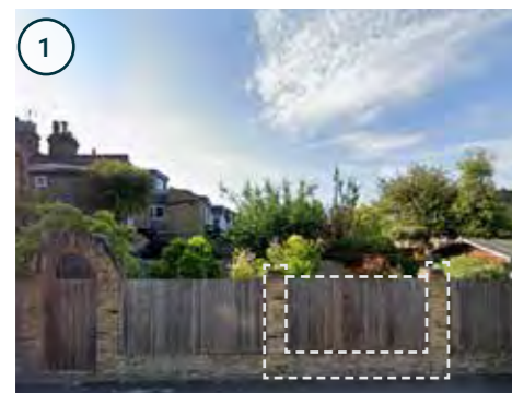
Wooden fence on brick piers
