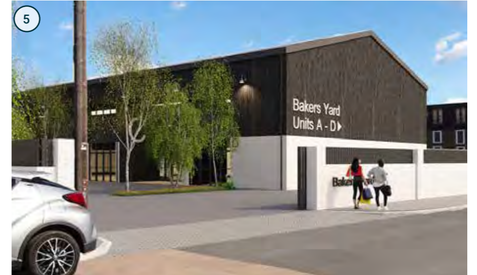
Dark timber cladding with white painted brick base
