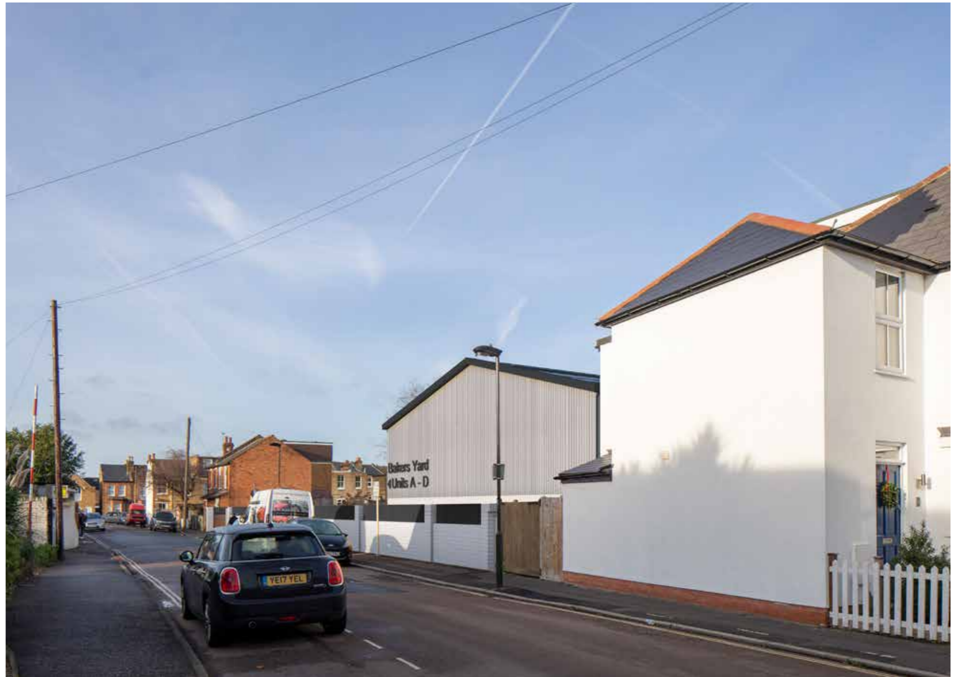
View west along Edwin Road
