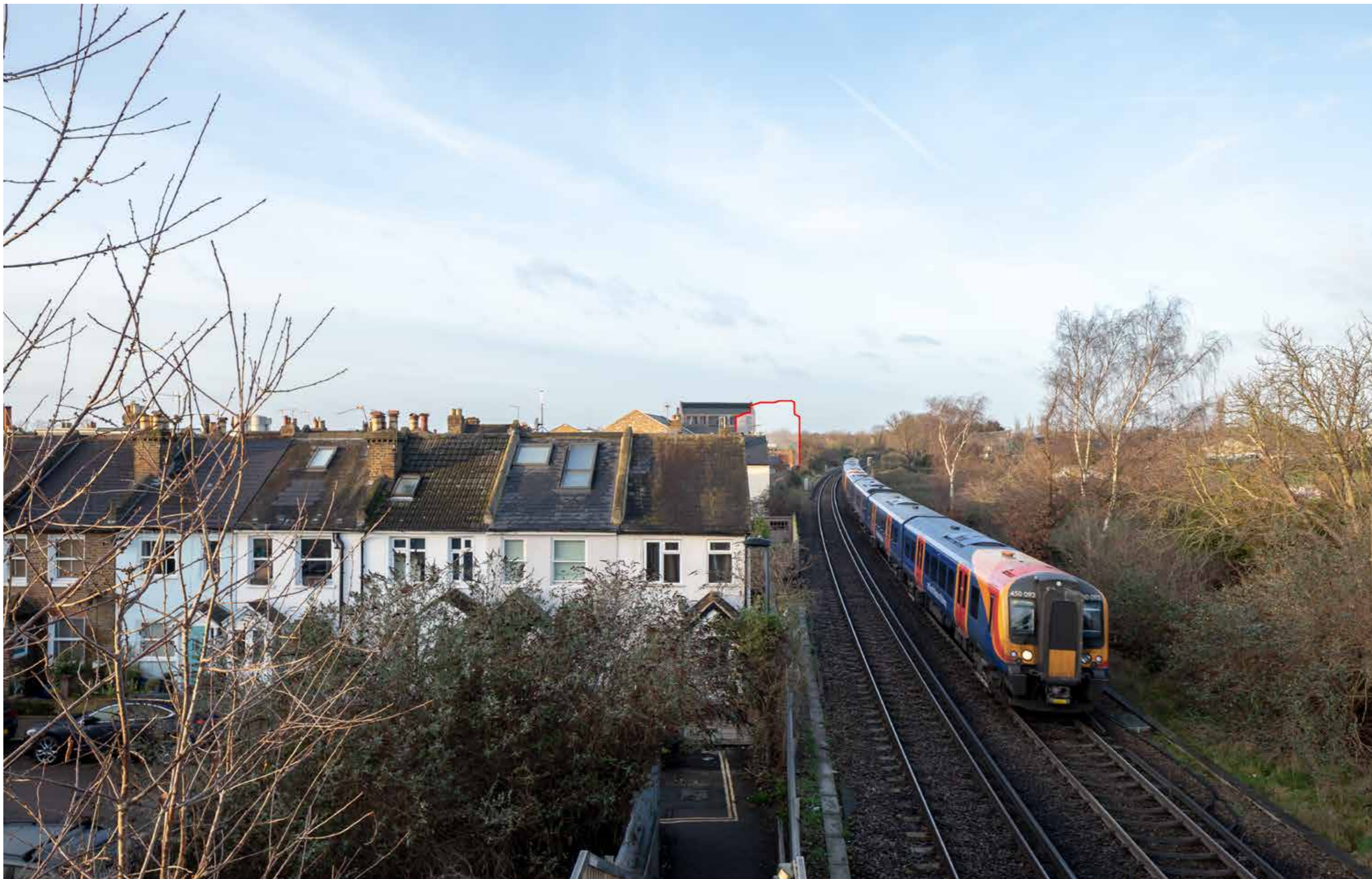
7. Footbridge crossing the railway, looking south west
