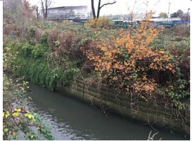
Photo 12: River Crane to the north of the site reinforced with concrete sides
