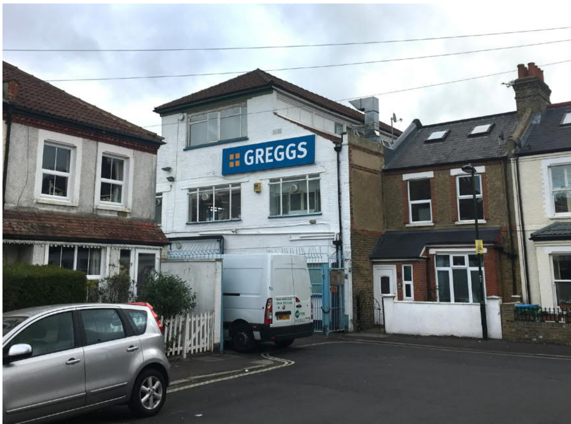
Figure 3-3: Existing access on Crane Road/Gould Road
