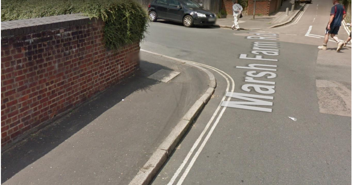
Figure 1-3: Tyre marks on Marsh Farm Road footway
