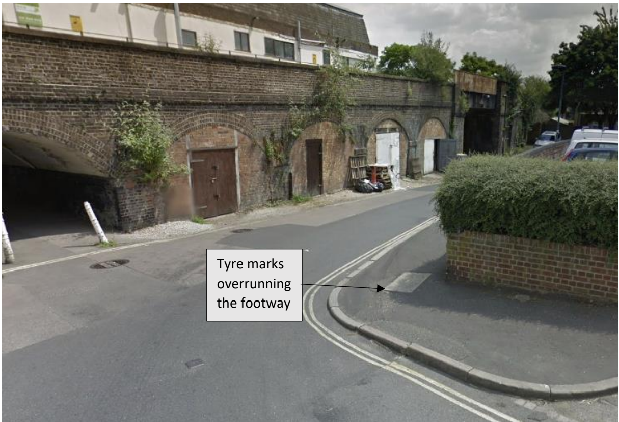
Photo 5: Tyre marks on Marsh Farm Road footway and Public Right of Way (PROW)
