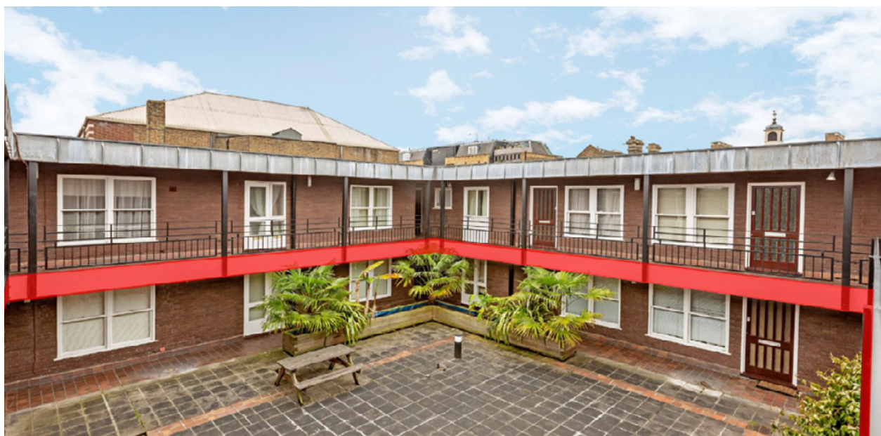
Figure 07: Overhanging Walkway Removed for 'No Balconies' Assessment
