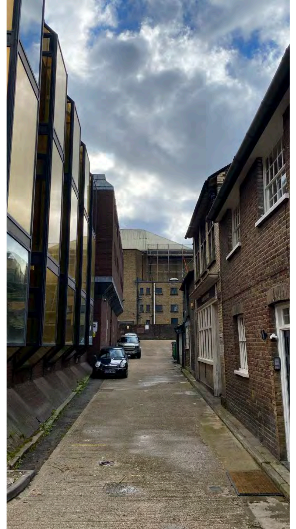
5. BOH of Hill Street Retail and Restaurant - Current Castle Yard Car Parking Area
