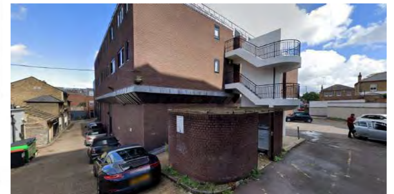
F : Castle Yard Repave in concrete setts with subtle marking for accessible parking bays.
