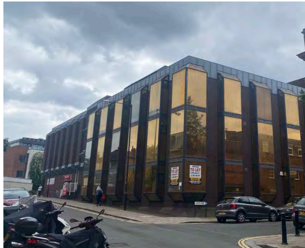
1. Lewis Road View - Current Building Outlook
