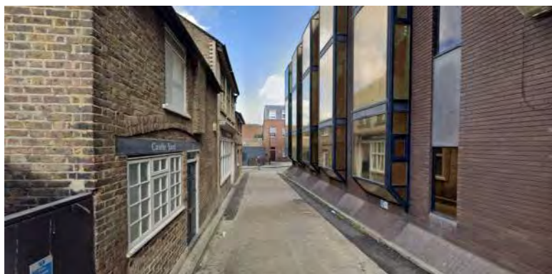
C : Castle Yard Repave in concrete setts - from building edge to building edge to provide consistent and shared surface.
