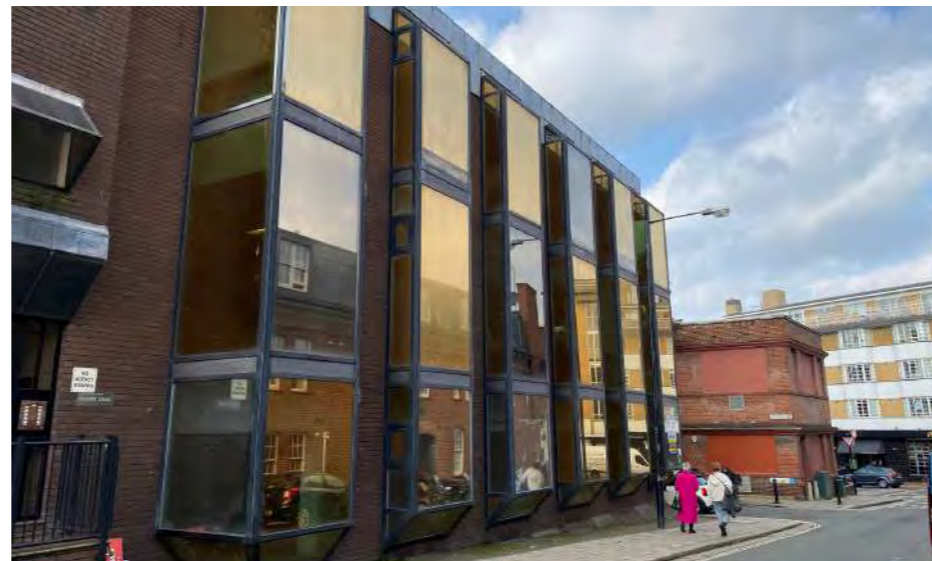
3. View from Lewis Road
