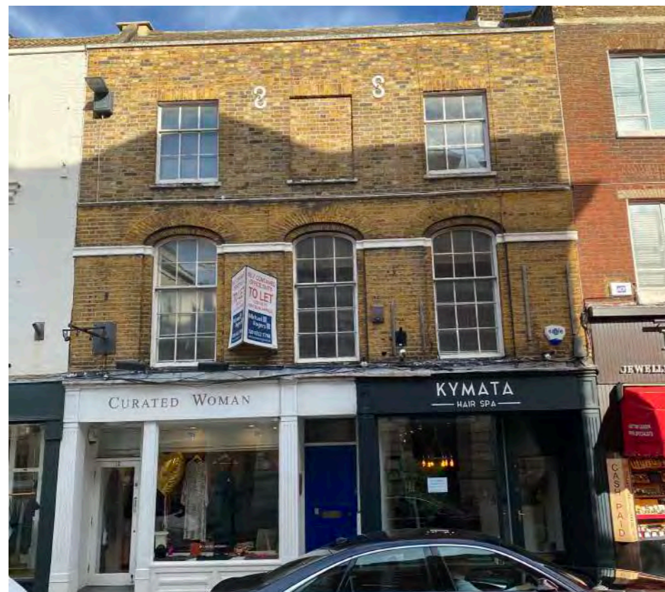
3. 12 & 14 Hill Street, Grade II listed building
