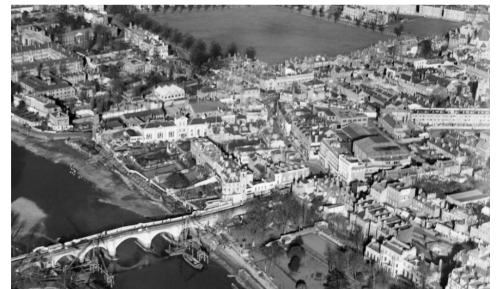
6. 1937 Richmond Bridge and Surrounding
