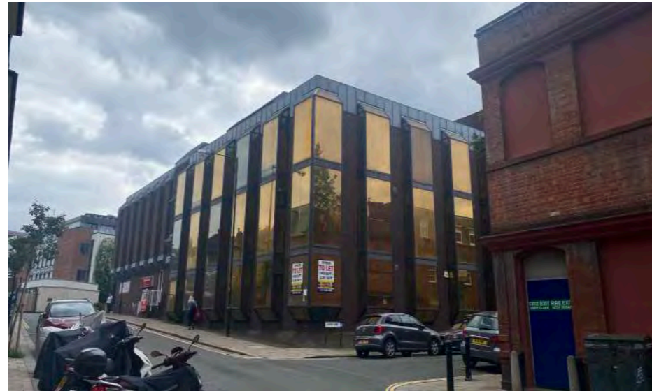
1. View from Lewis Road
