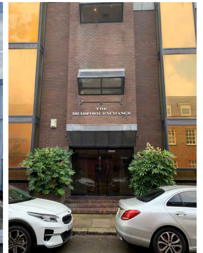
6. Current Stepped Entrance - No disabled access
