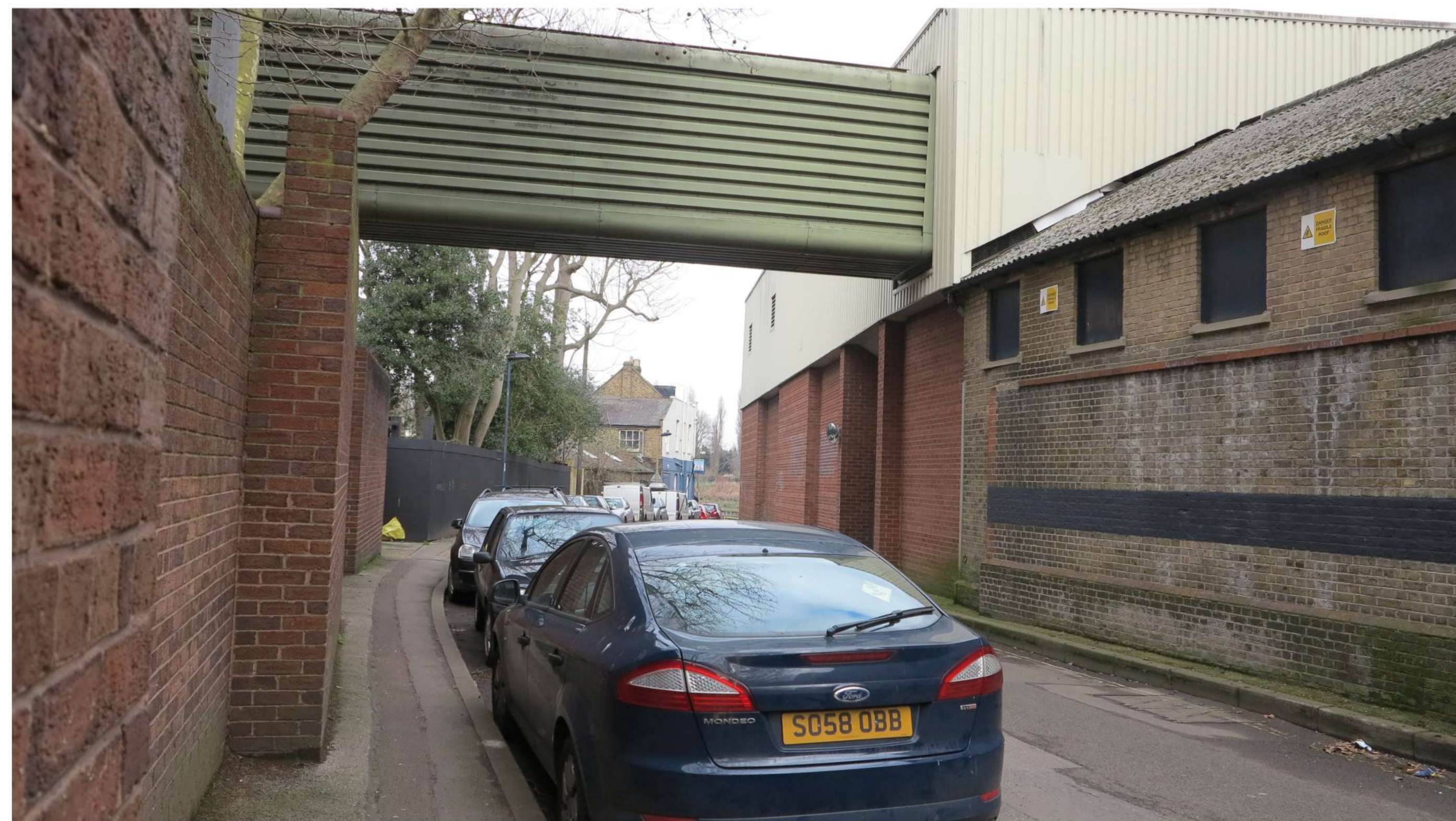
Photograph of Ship Lane looking north east showing existing buildings above.
