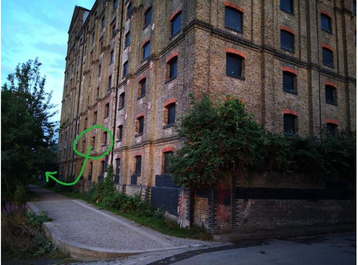
Plate 1 – 2019 Soprano pipistrelle emergence location from a second-floor window on the northern façade of The Maltings (B8).
