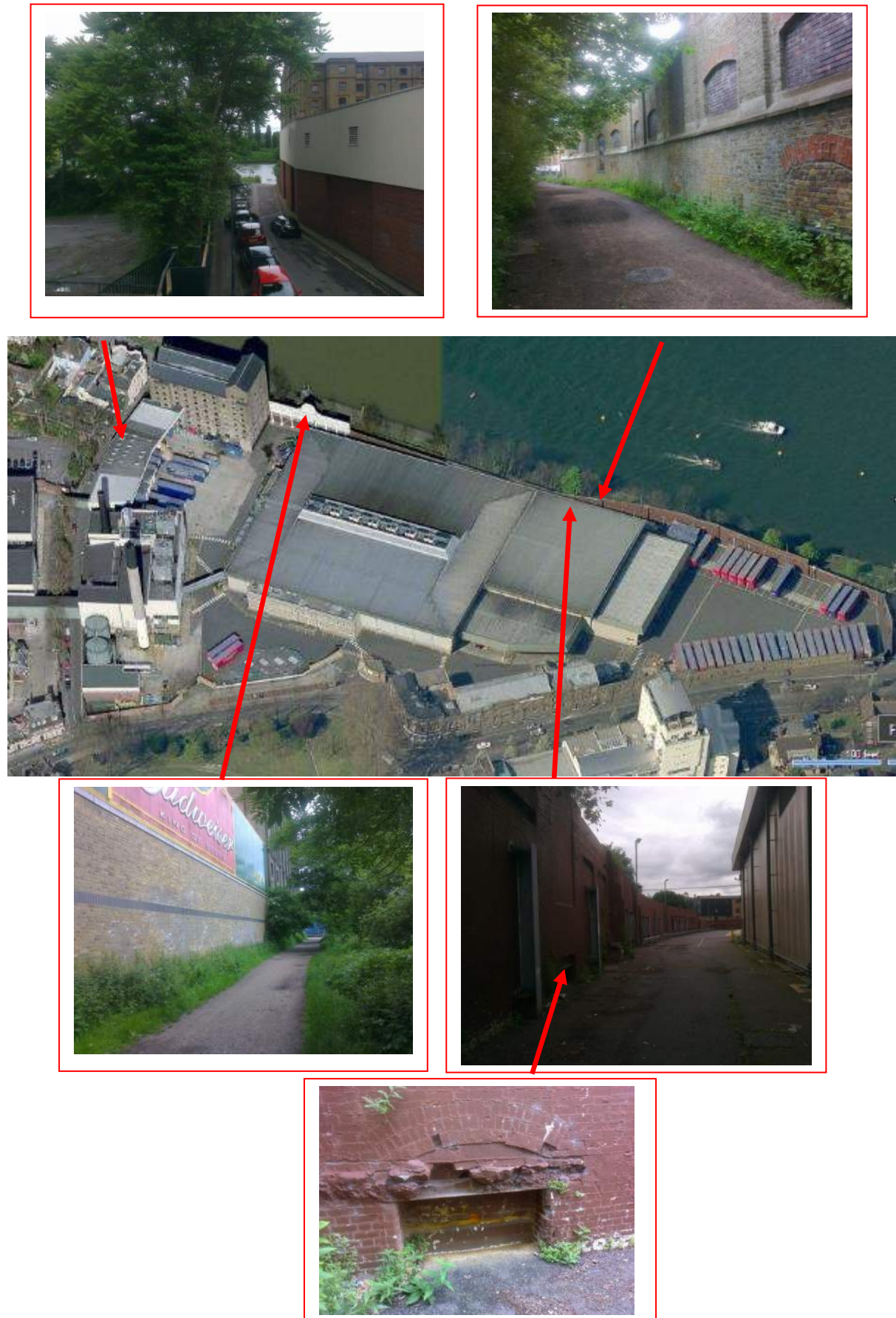
Figure 4-4 The extent of existing tidal defences
