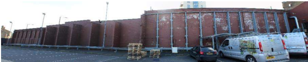
Plate 29 Internal elevation of south boundary wall (2017)
