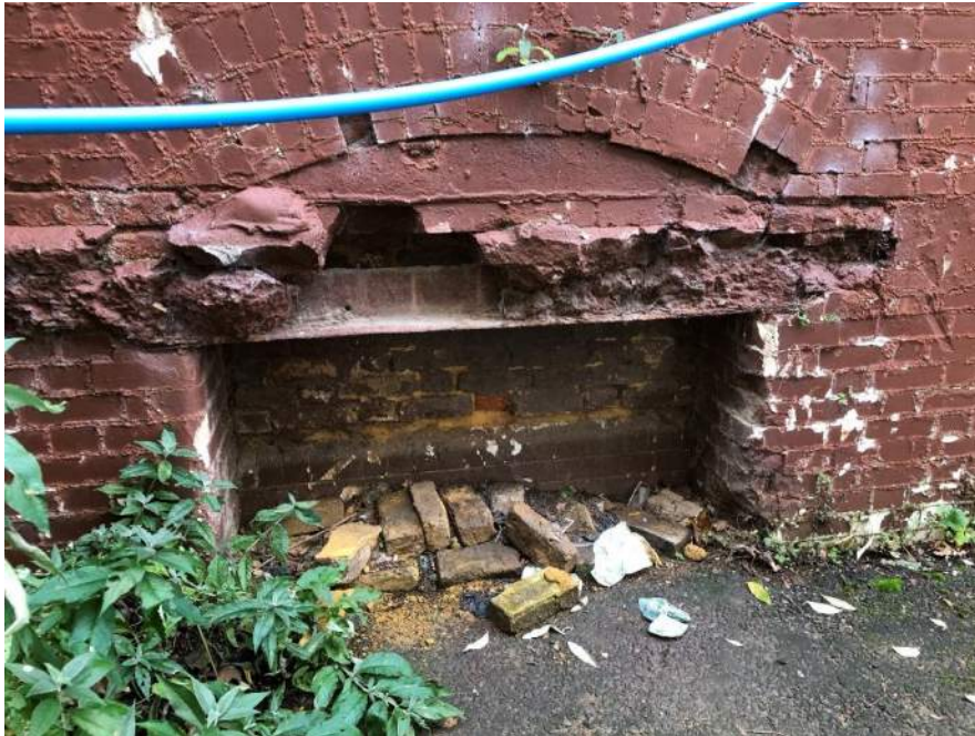
Plate 26: Interior elevation of north boundary wall (2021)
