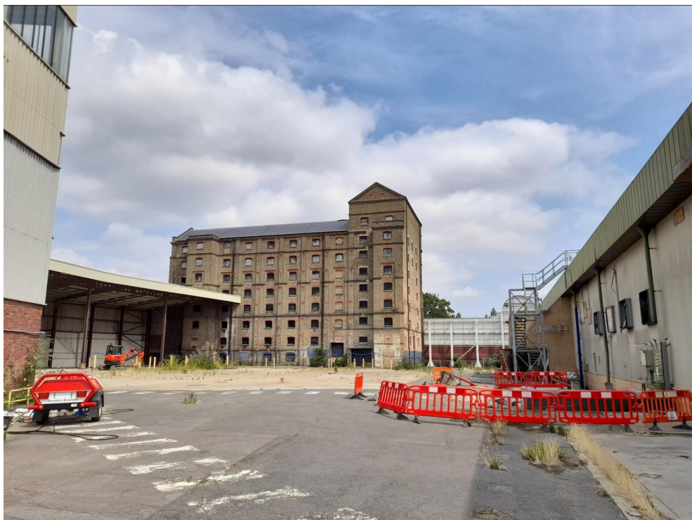
Plate 11: Section of northern boundary wall (HA004) to the right of the maltings building (HA003), viewed from within the site. Existing view to north
