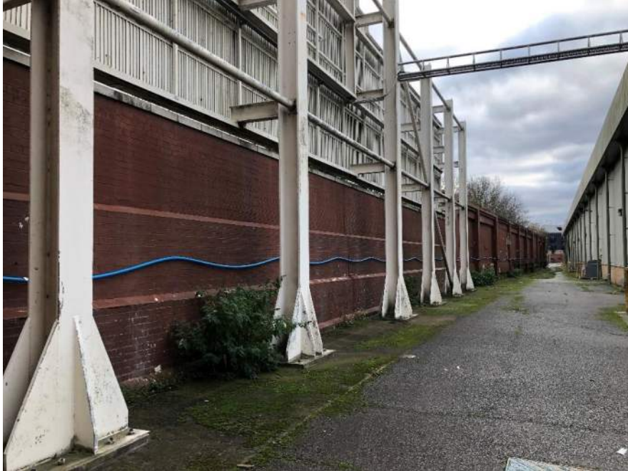
Plate 24: Interior elevation of north boundary wall (2021)
