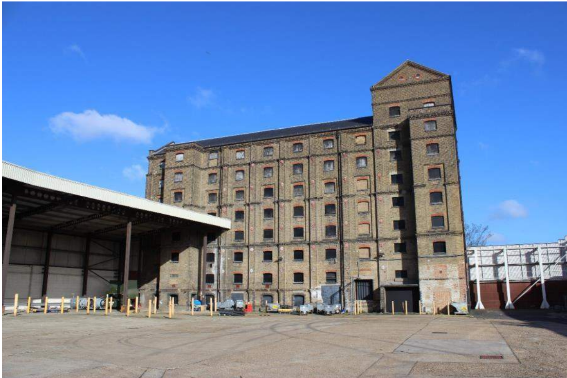
Plate 11: South facing elevation of Maltings (2017)
