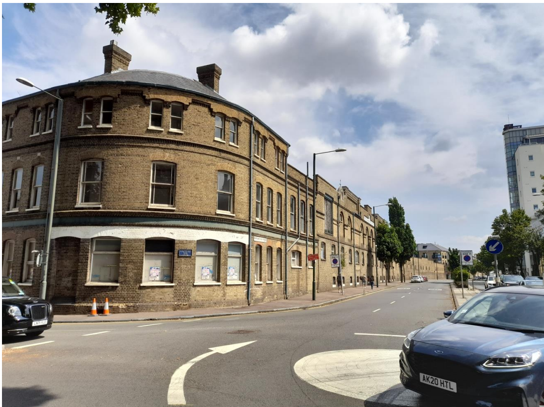
Plate 1: Former hotel and bottling buildings and southern boundary wall. Existing view to east
