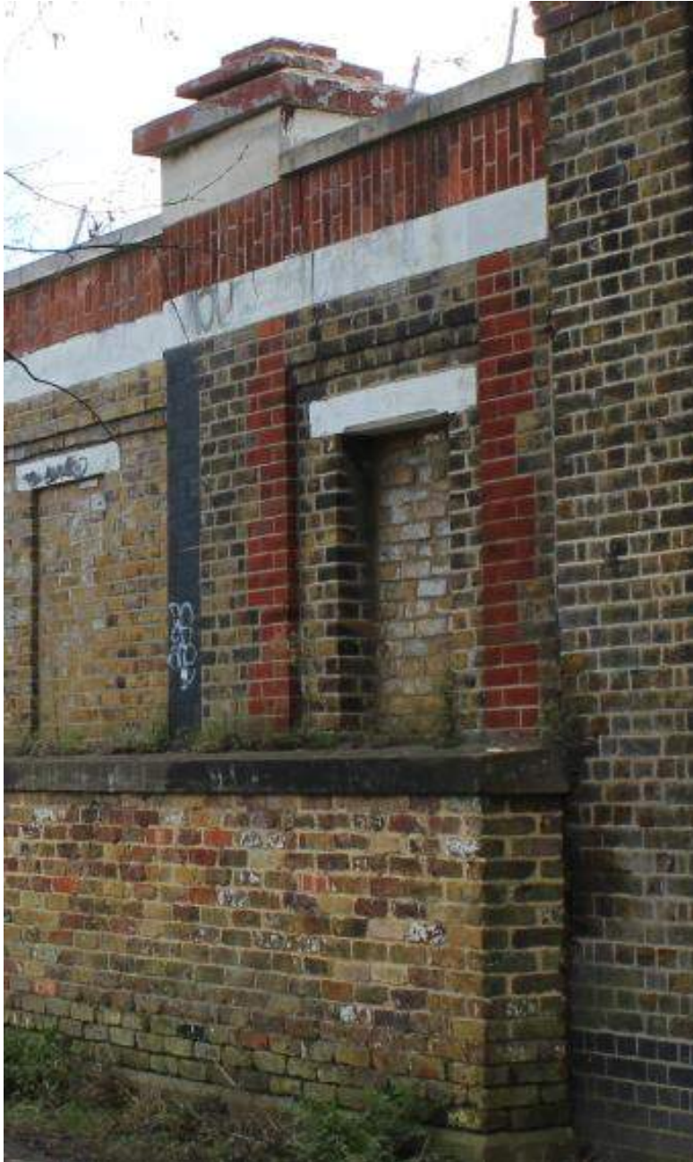
Plate 20: Section 5 - including gate pier (2017)
