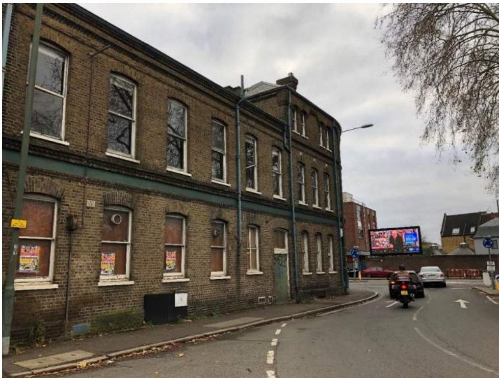
Plate 2: West facing elevation of Former Hotel (2021)
