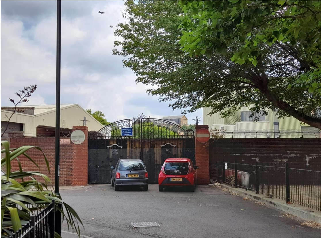
Plate 12: Historic gates on William's Lane with the maltings building visible in the background. Existing view to north-east
