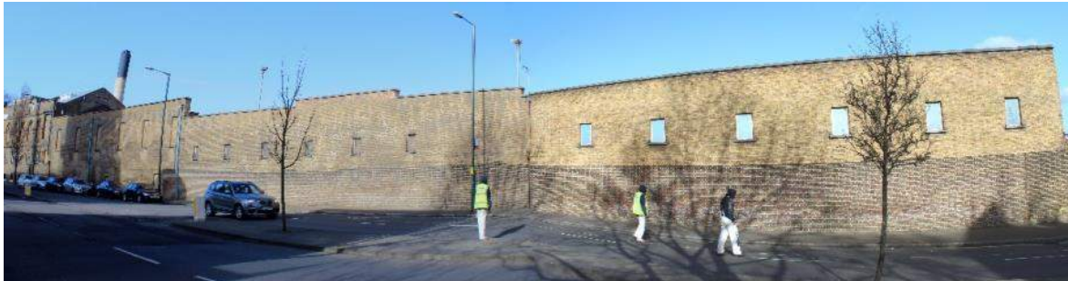
Plate 28 External elevation of south boundary wall with section 1 (left end) and section 2 (right end) (2017)
