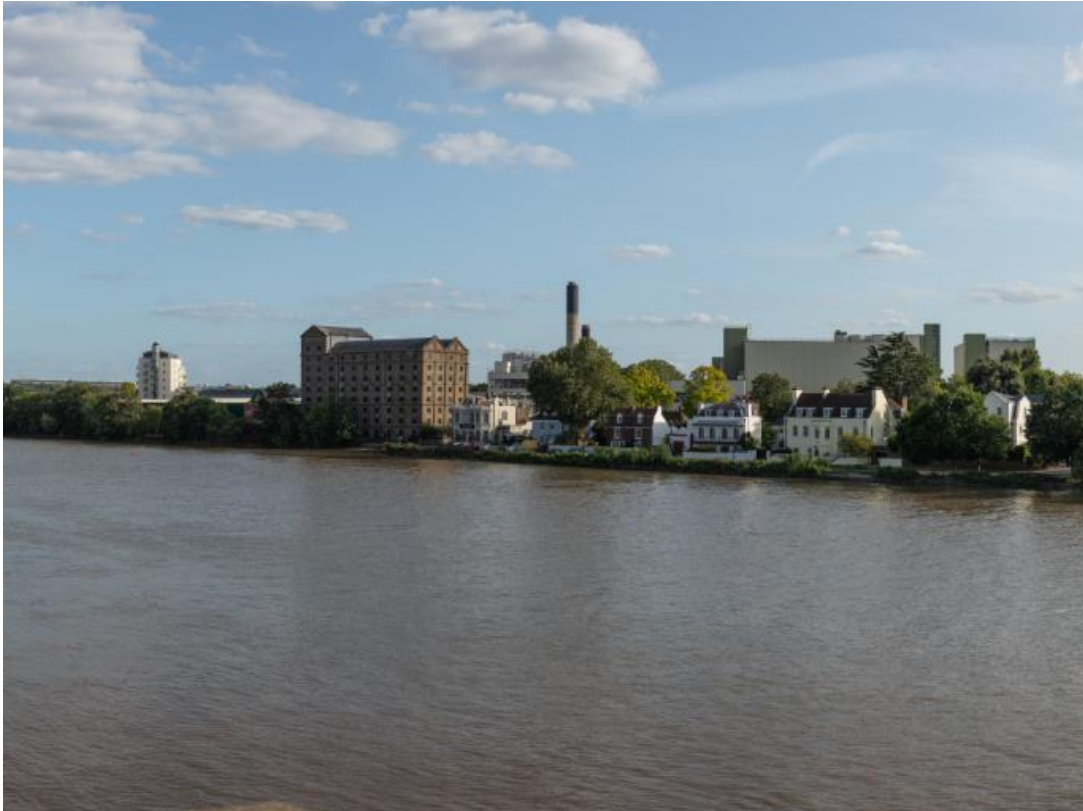
Plate 3: View towards the maltings building from Chiswick Bridge. Existing view to south-east
