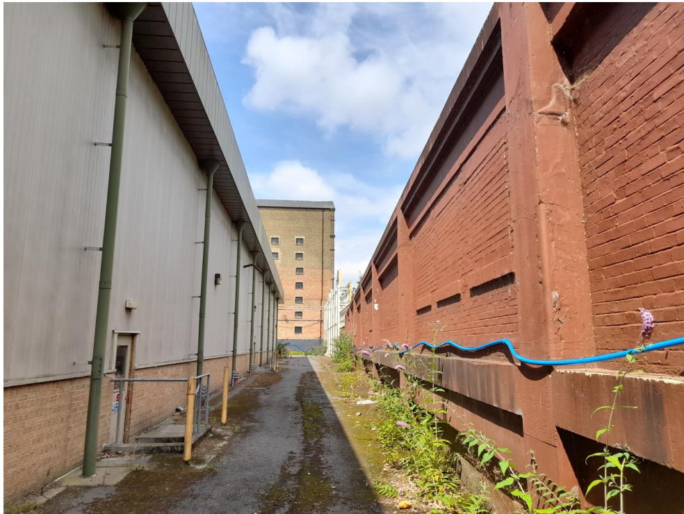
Plate 10: Section of northern boundary wall (HA004) adjacent to the maltings building (HA003), viewed from within the site. Existing view to west.
