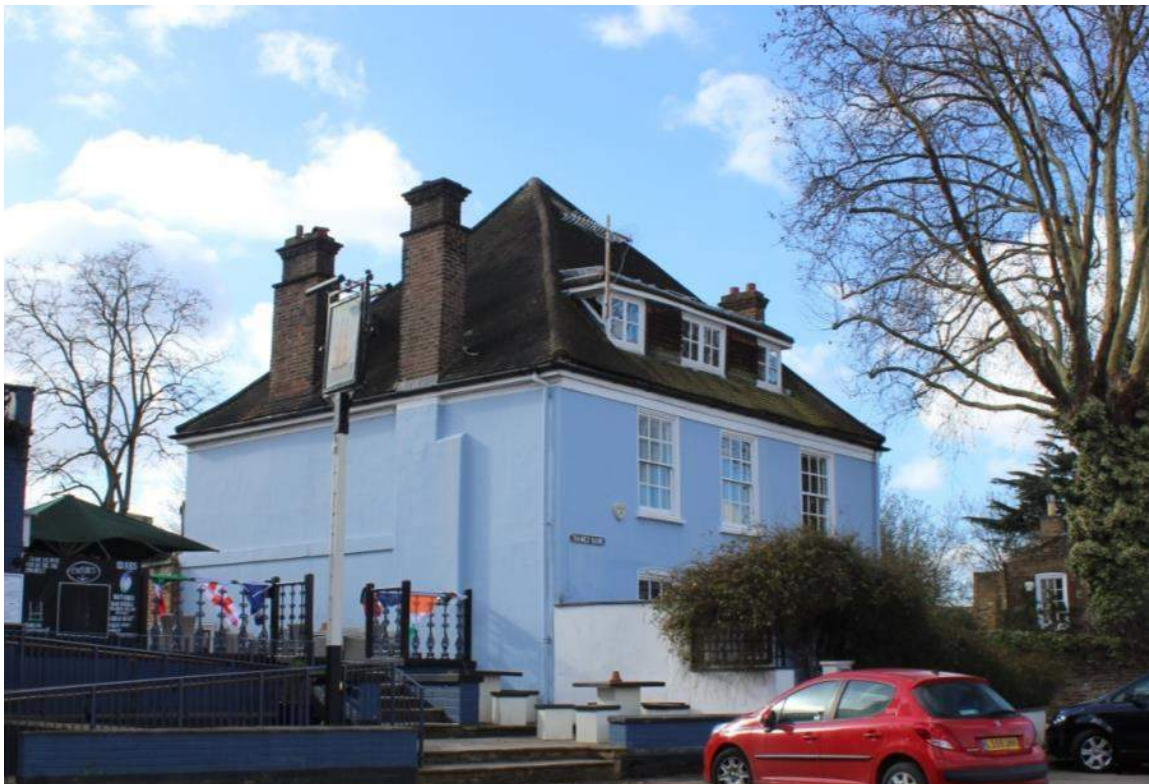
Plate 37: Grade II Listed Thames Cottage (2017)
