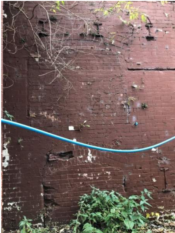
Plate 25: Interior elevation of north boundary wall (2021)
