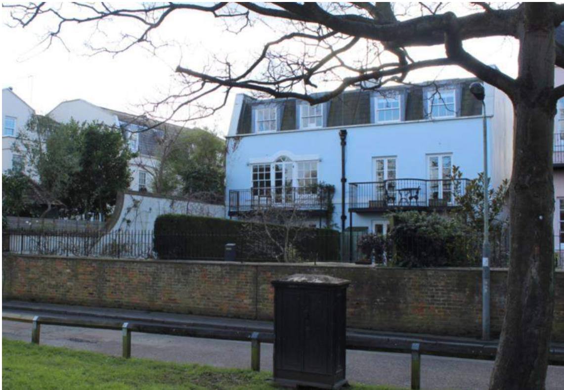
Plate 39: Building of Townscape Merit 6 and 7 Thames Bank (2017)
