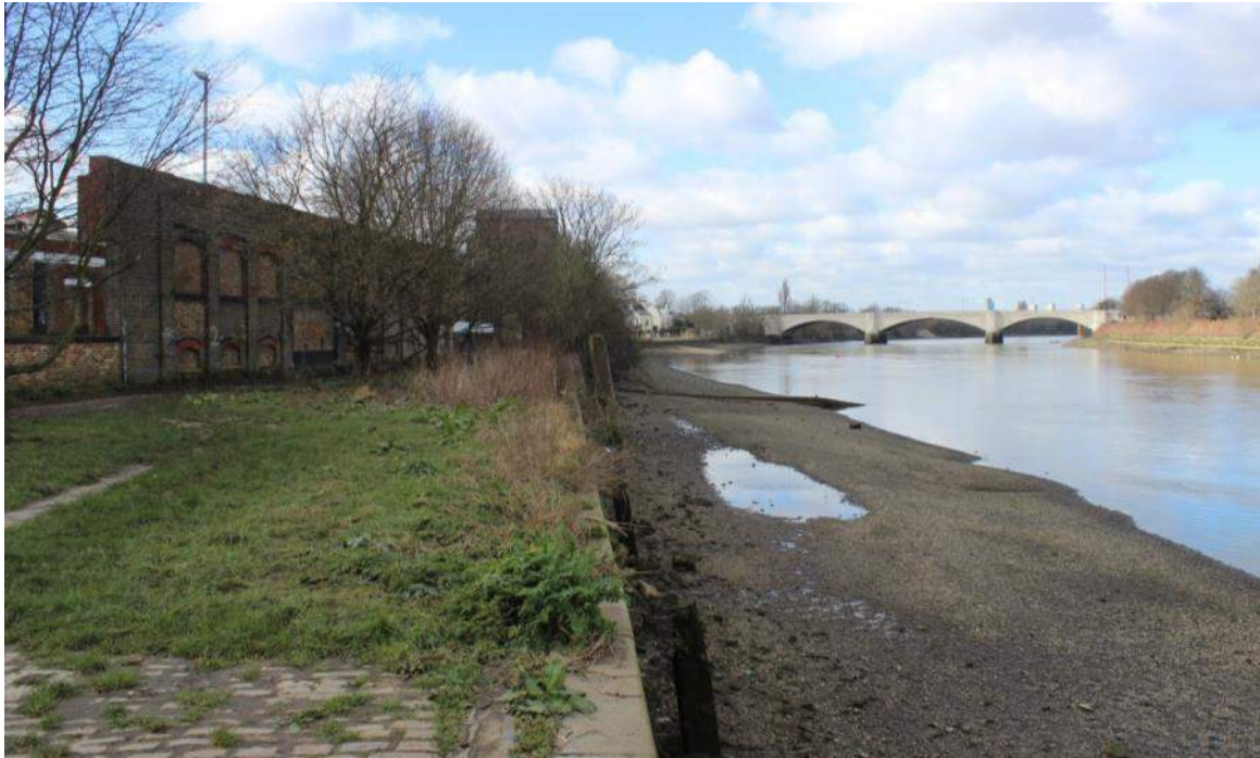
Plate 32: Timber river moorings along the riverside (2017)
