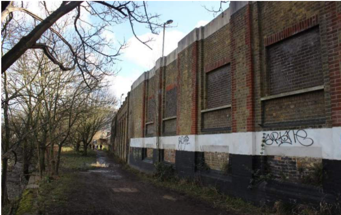
Plate 18: Section 3 - Wall of 1937 Tun Block
