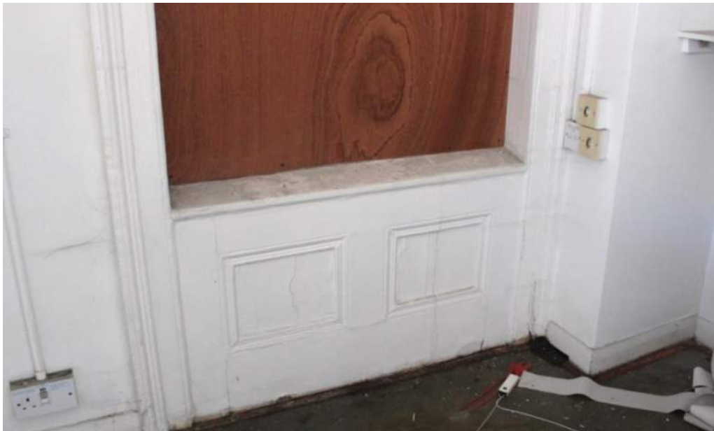
Plate 4: Surviving timber panelling to interior of Former Hotel (2017)
