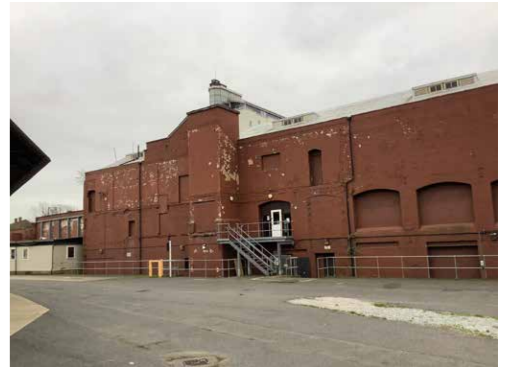
Former hotel and canteen building at brewery West Site
