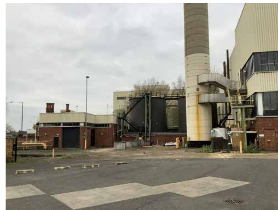
Remaining tanks south of Energy Centre at brewery East Site
