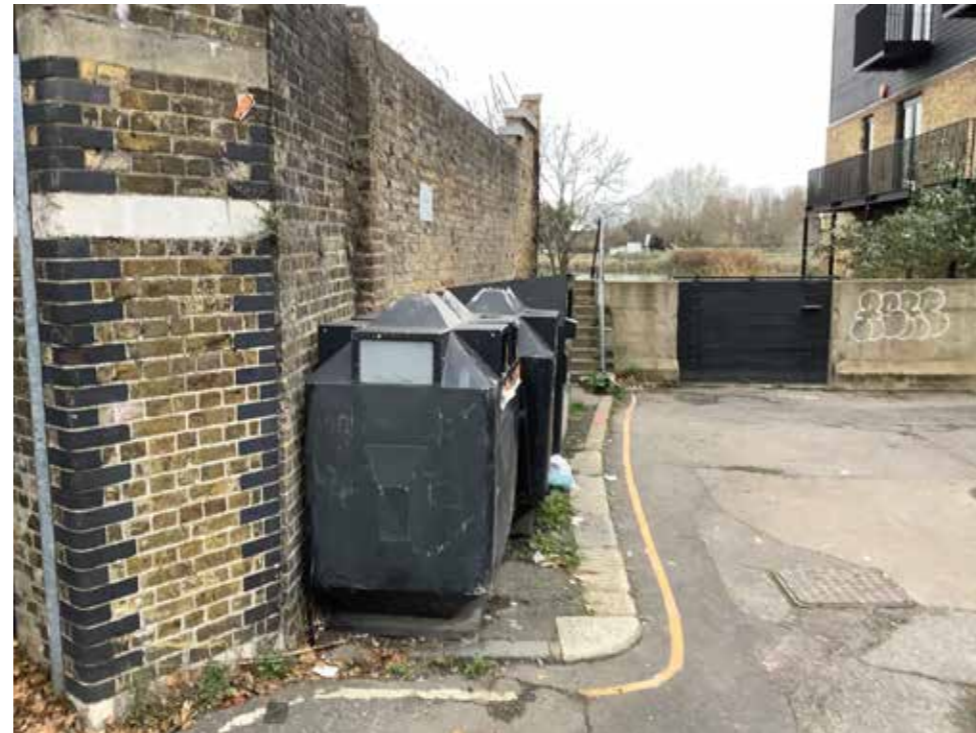
Off-site existing flood defence east of the Site
