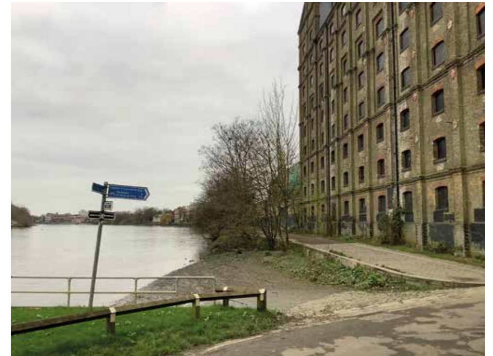
North Project Boundary with River Thames
