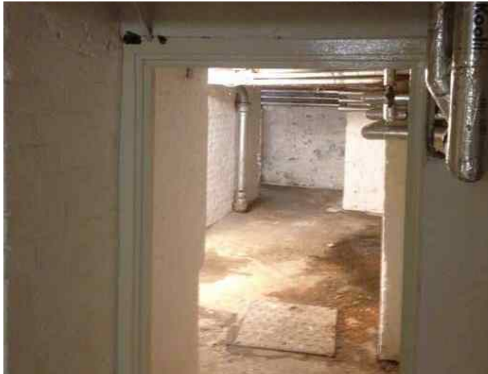
The (former) Hotel cellar used as the staff canteen
