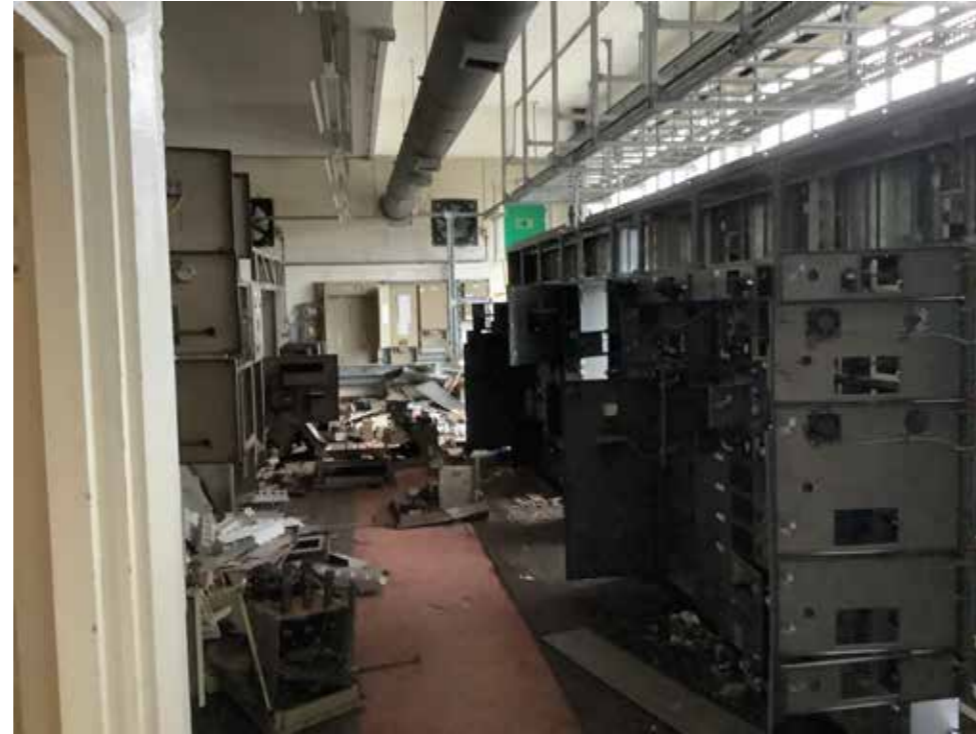
Residual electrical cabinets following strip out of Energy Centre
