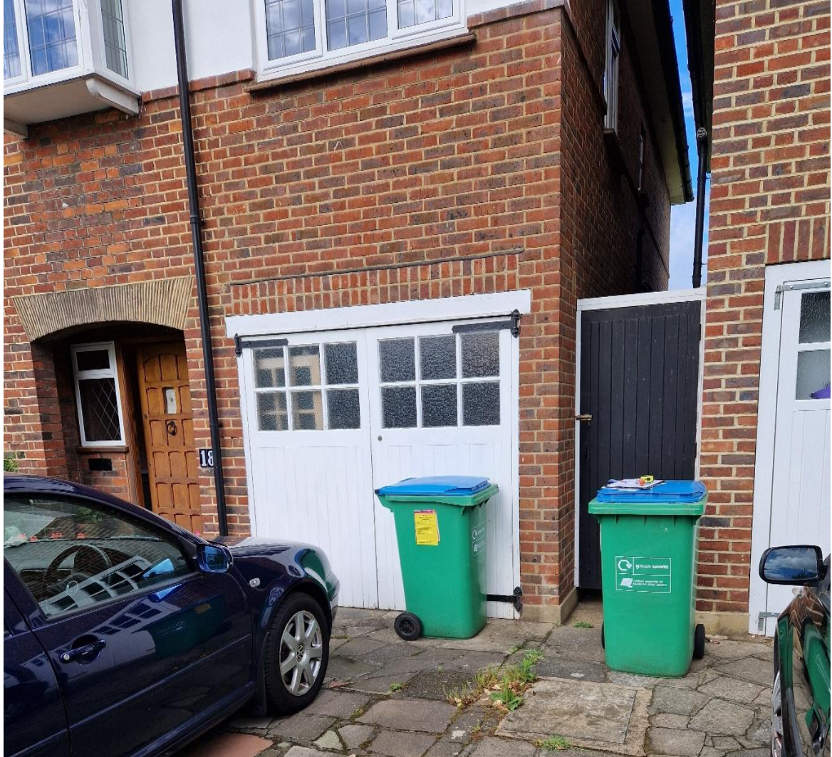
Fig 1.2. View of Front (East) Elevation Showing Garage Doors
