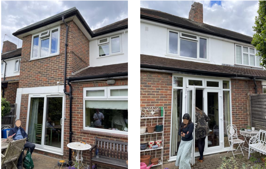
Fig 1.3. View of Rear (West) Elevation
