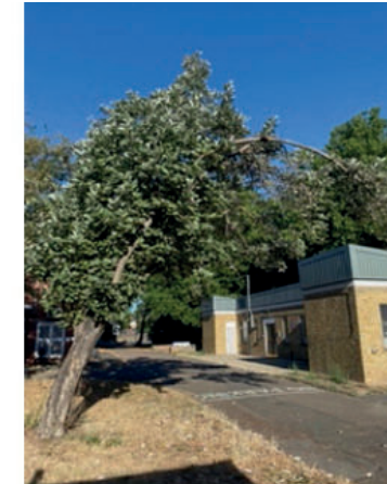
Storm damaged Whitebeam, T63 now further unbalanced
