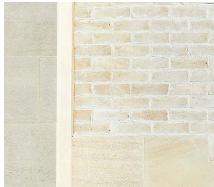
Buff Brick and pre-cast banding
