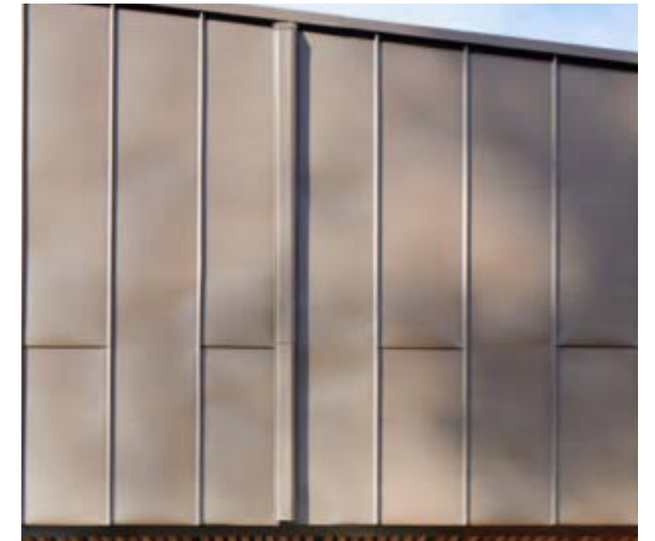
Standing seam metal cladding
