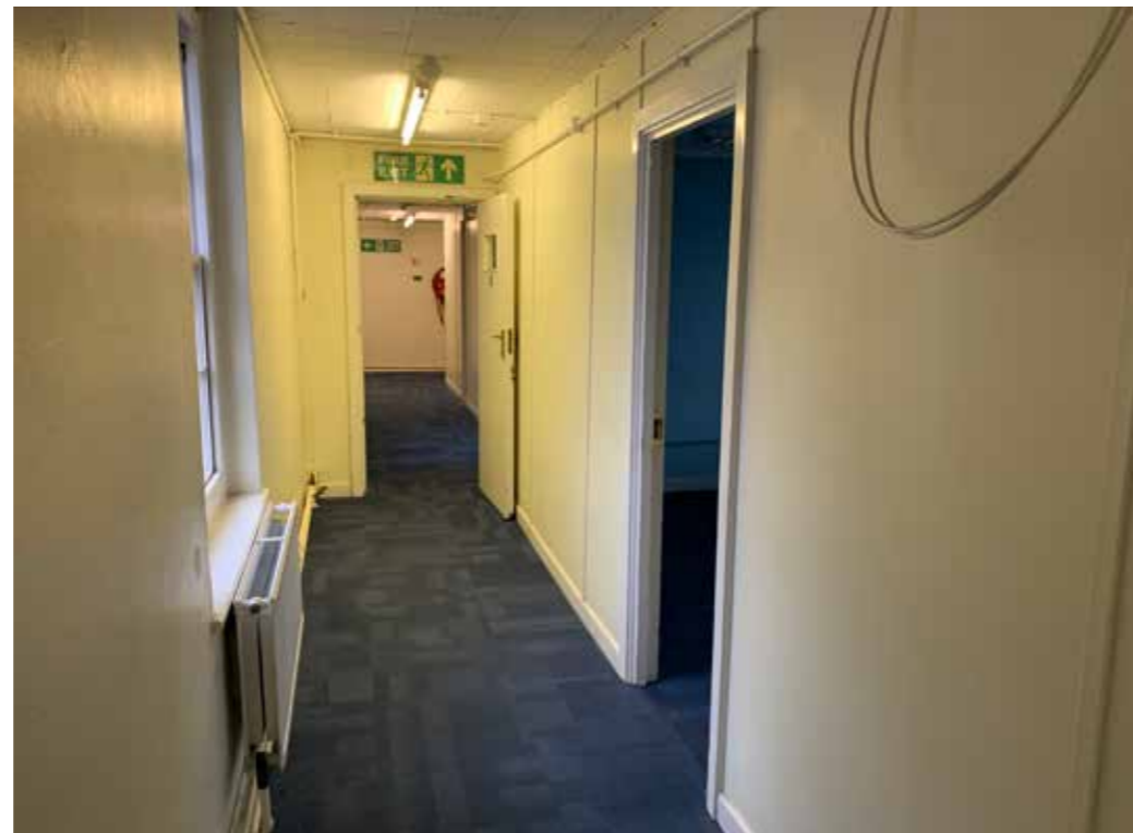
Figure 4.26 Modern partition walls have been introduced into the west wing to create corridors
