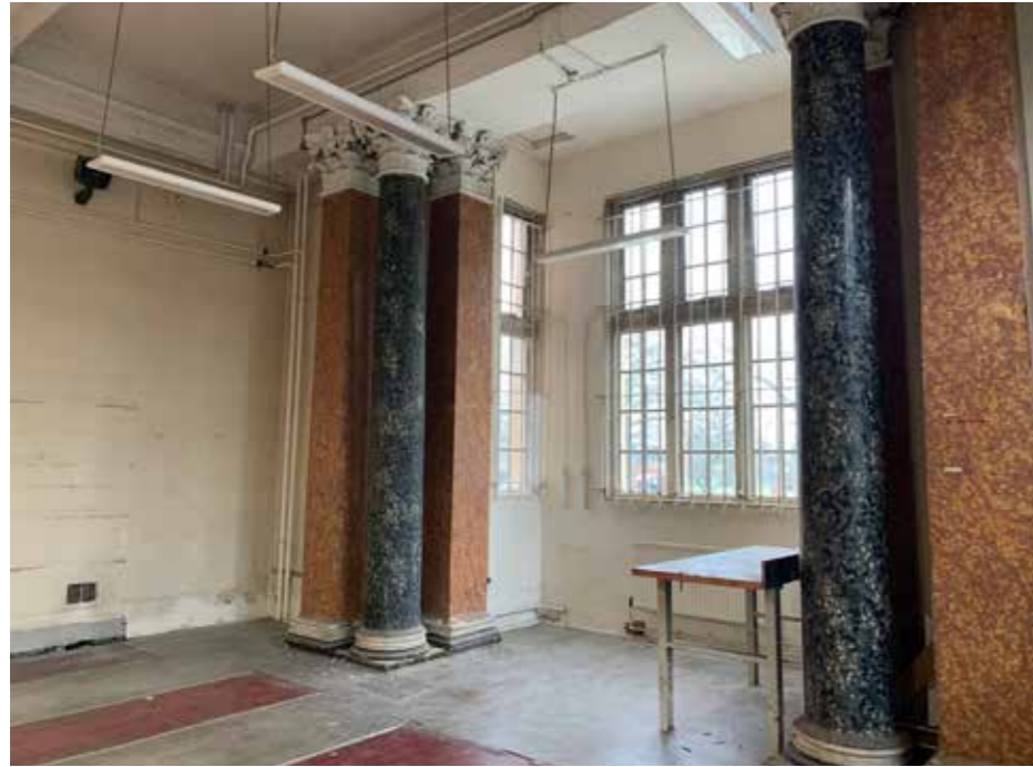
Figure 4.12 Columns, believed to be the 'scagliola columns' identified by the 1841 survey, survive in their early-eighteenth century situation in the east wing. Alterations to the room have resulted in their awkward interaction with the alternating ceiling level.
