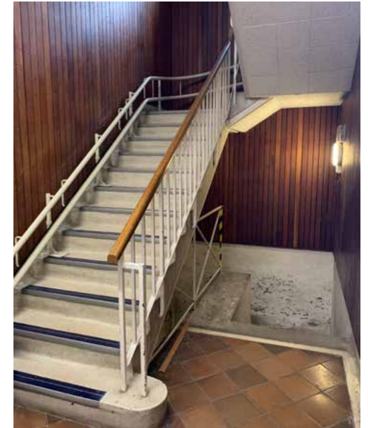
Figure 4.11 A staircase hall located on the east side of the building. Its staircase comprises modern fabric with a plain design and its walls have been covered by timber panelling
