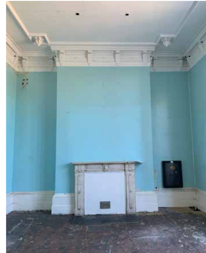
Figure 4.19 Where historic decorative features survive in situ, such as this fireplace, cornicing and ceiling moulding, they provide a principal source of interest
