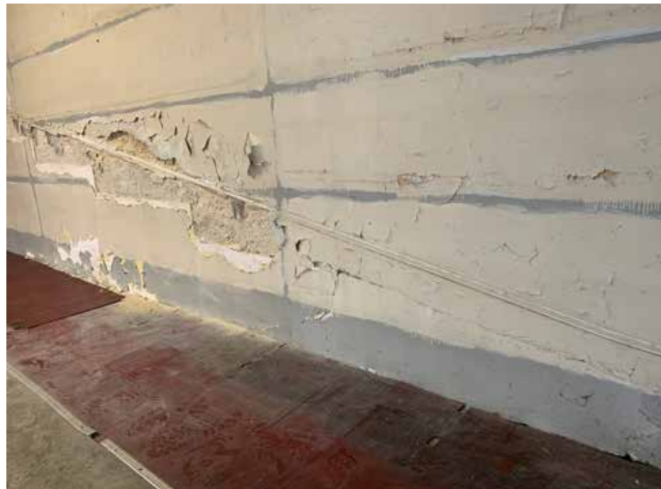
Figure 4.13 Elements of chasing within plastered walls of the front, eastern classroom reveal the position of historic tiered seating
