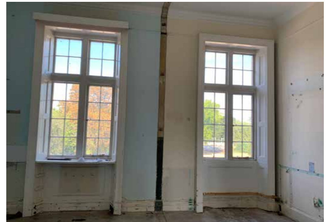
Figure 4.24 A detractive, modern partition has been removed as part of consented enabling works. This exemplifies how the removal of such partitions can reinstate the historic volume of spaces and enhance their significance
