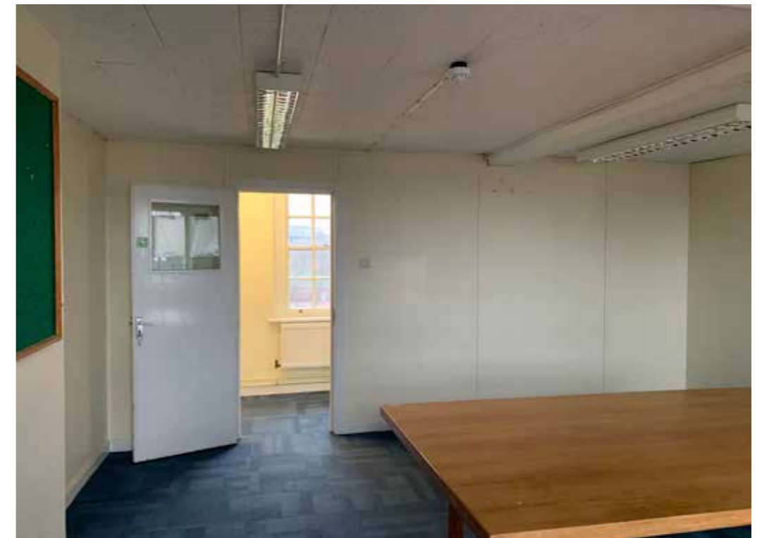
Figure 4.28 Modern finishes typically installed within rooms located in the west wing include partition walls, suspended ceilings, light fixtures, doors and carpet
