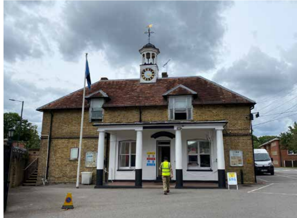
Figure 4.29 The Guardroom, located west of the hall
