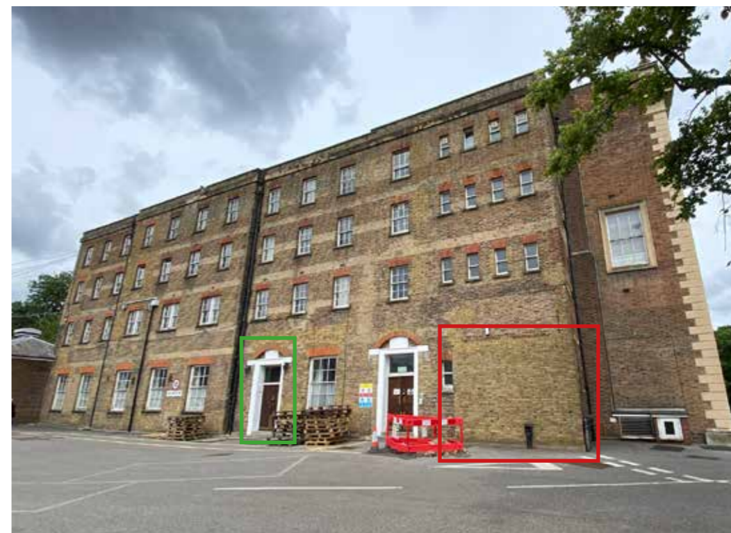
Figure 4.4 The west service wing of the building has experienced extensive alteration to its fenestration and general facade. Red = evidence for a former extension to the elevation. Green = an existing, non-historic entrance has been created through the adaption of an original window.
