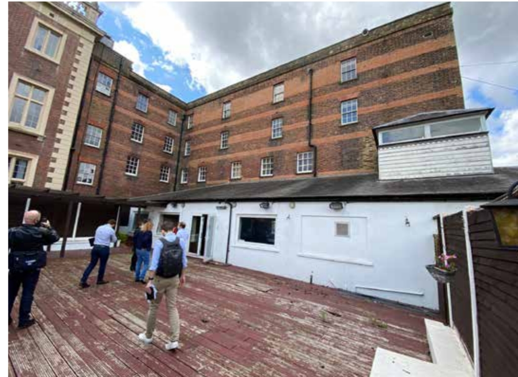
Figure 4.3 Rear north elevation of the hall, showing the new central range designed by George Mair (left) and the early-nineteenth century service wing (right). The rebuilt 'covered way' is shown in the foreground and the twentieth-century staircase tower is also visible.
