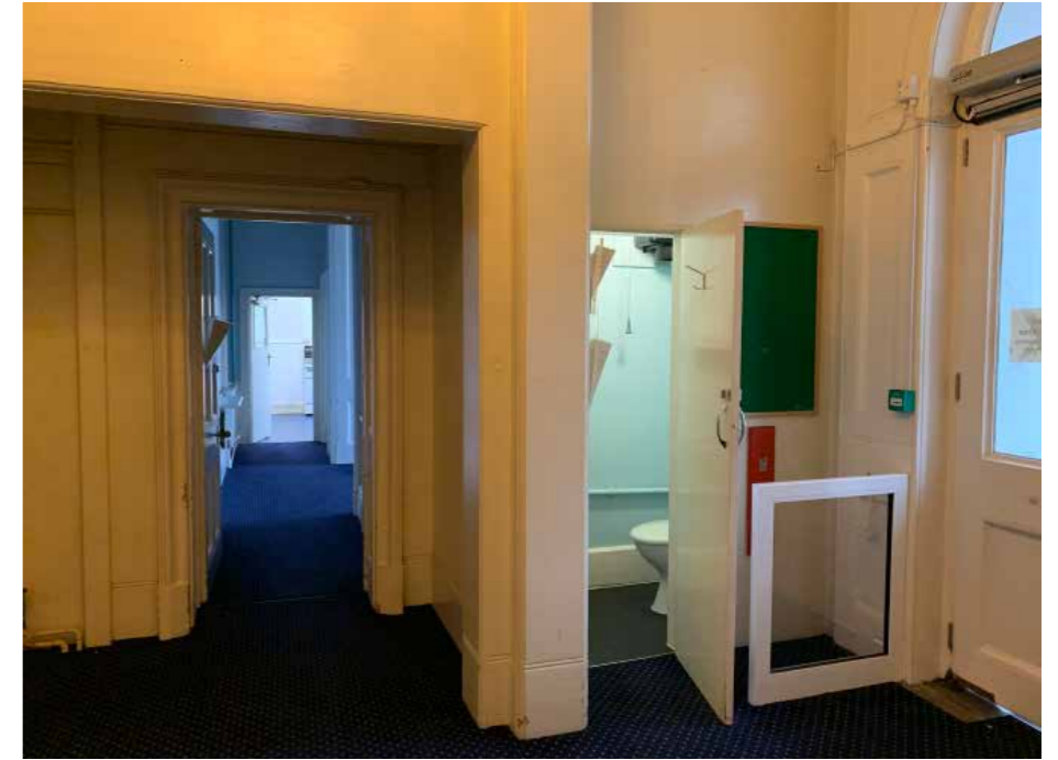
Figure 4.16 The plan of the rear entrance hall has been much altered by the blocking up and creation of new openings.
