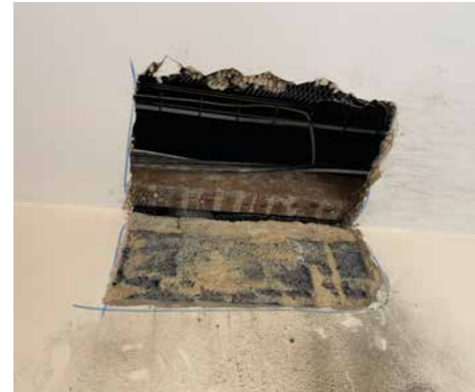
Figure 5.13 Photograph of the heavy block wall build up amongst existing walls within the west wing at second floor level which are proposed to be removed Drawing produced by ADP Architecture
