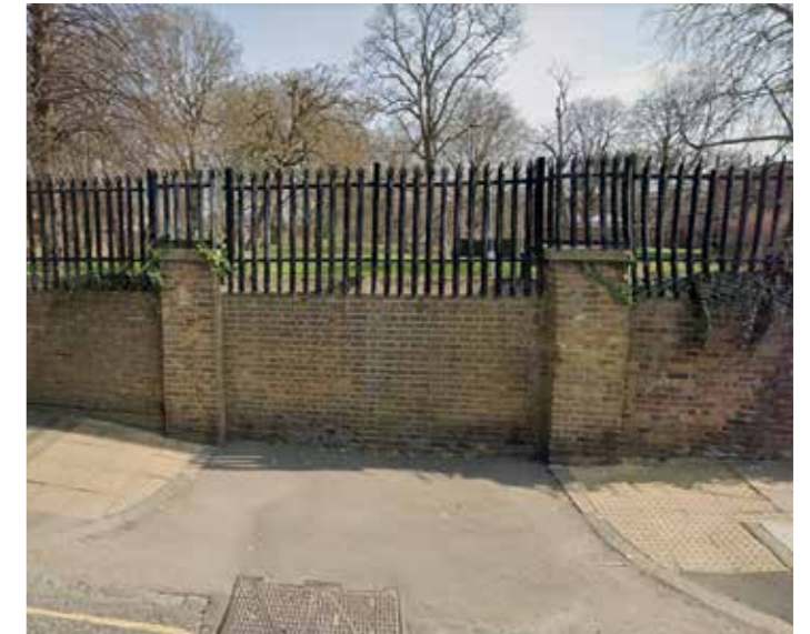
Figure 5.3 Photograph of the existing blocked gate entrance on the west boundary wall of the Site
