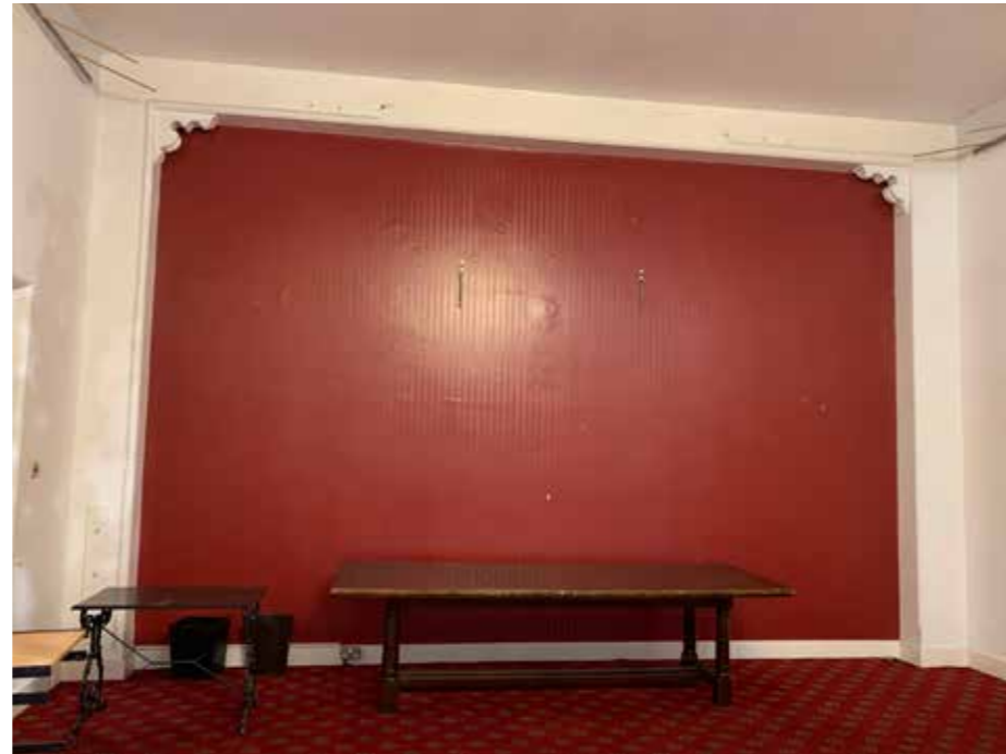
Figure 4.14 The north wall to the main entrance hall is possibly an original feature which has likely been altered by the construction of frame that supports the Chapel located above
