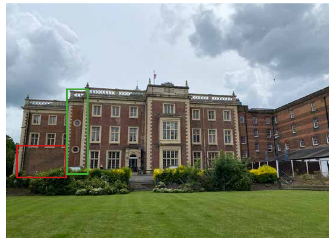
Figure 4.2 Rear north elevation of the hall. Red = exposed brickwork belonging to Hardwick's nineteenth-century wing. Discolouration in the brickwork indicates the location of a former staircase and terrace in this location. Green = a 1970s staircase tower which responds well to the architectural treatment of the hall's exterior.
