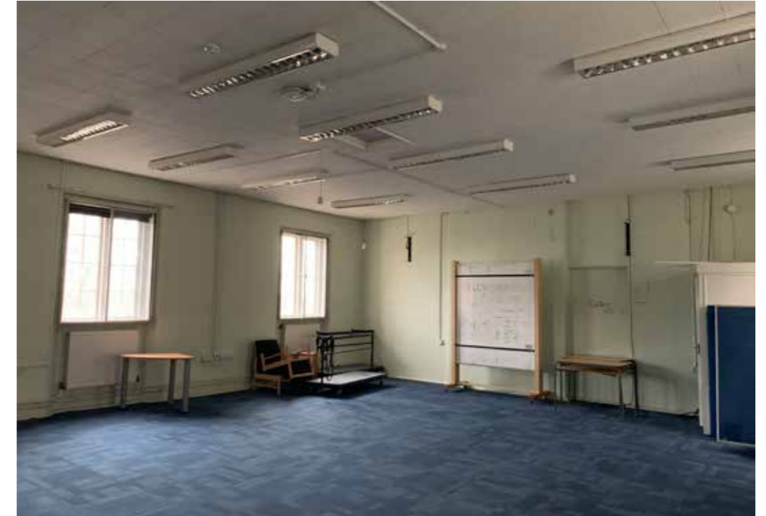
Figure 4.23 A modern dropped ceiling, window grills, carpet and electrical fixtures have been installed in a front classroom at second-floor level
