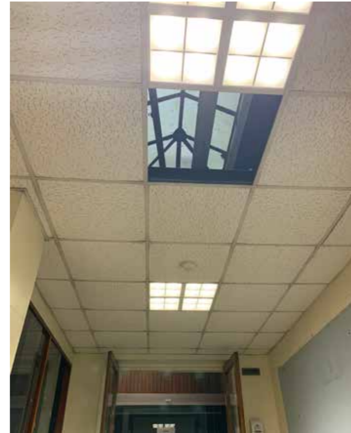
Figure 4.10 A modern dropped ceiling has been installed in the west-entrance corridor. It conceals the nineteenth-century skylight feature
