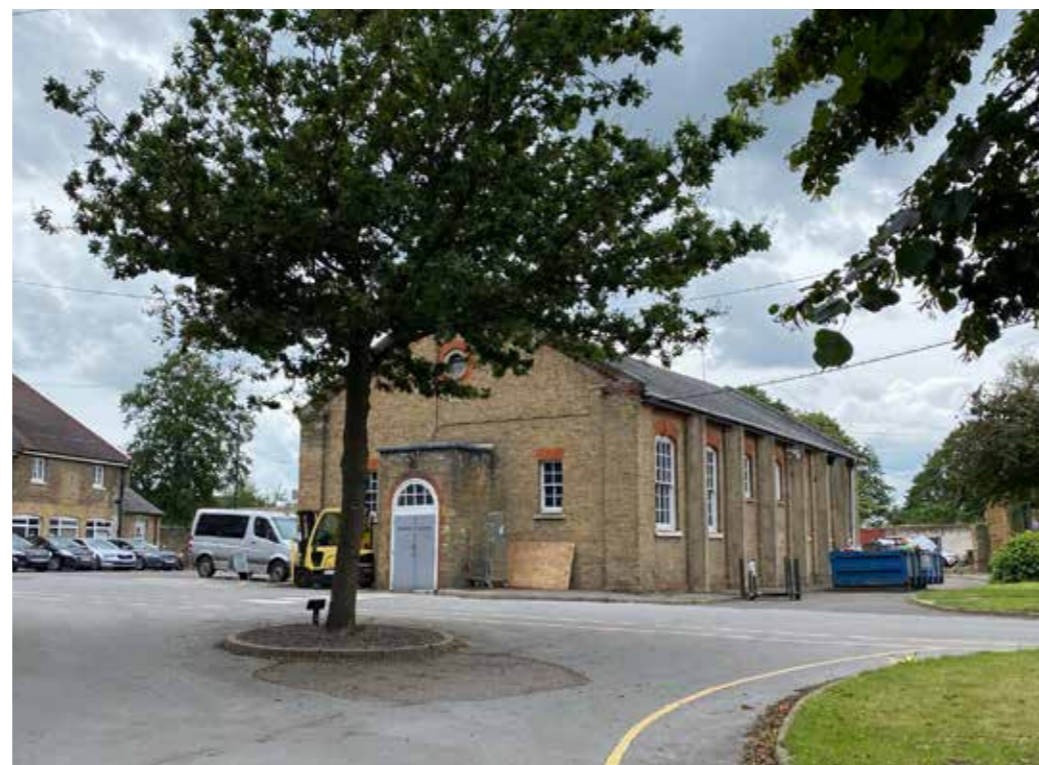
Figure 4.30 The Former Band Practice Hall is located west of the hall
