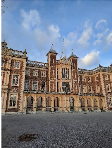
Plate 1: Front (south aspect) of building B0: Kneller Hall main building.
