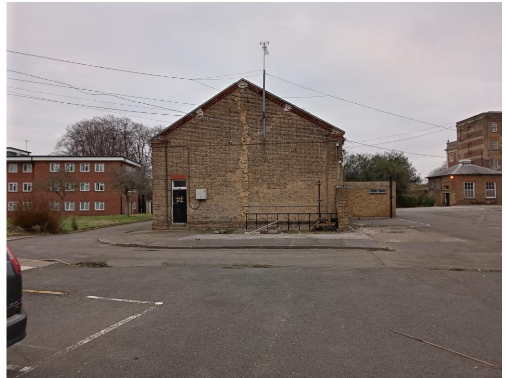
Photo 14: Grade II listed studio building taken from car park looking east. Stairs lead down to basement plant room.
