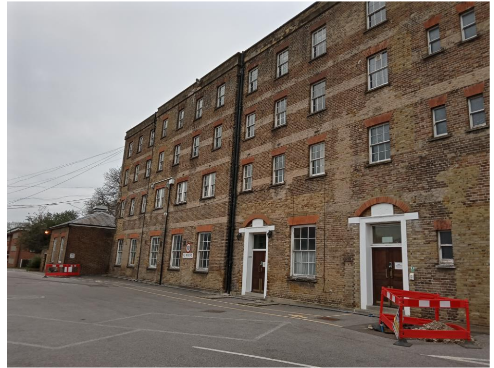
Photo 2: Western side of Kneller Hall with flat access into building.
