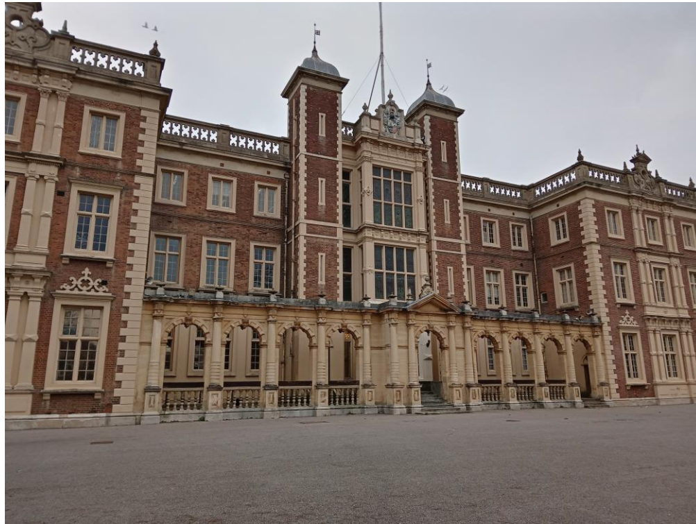
Photo 1: Overview of Kneller Hall from the south.
