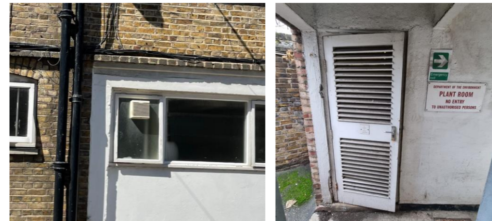
Fig 6. Existing building services elements
