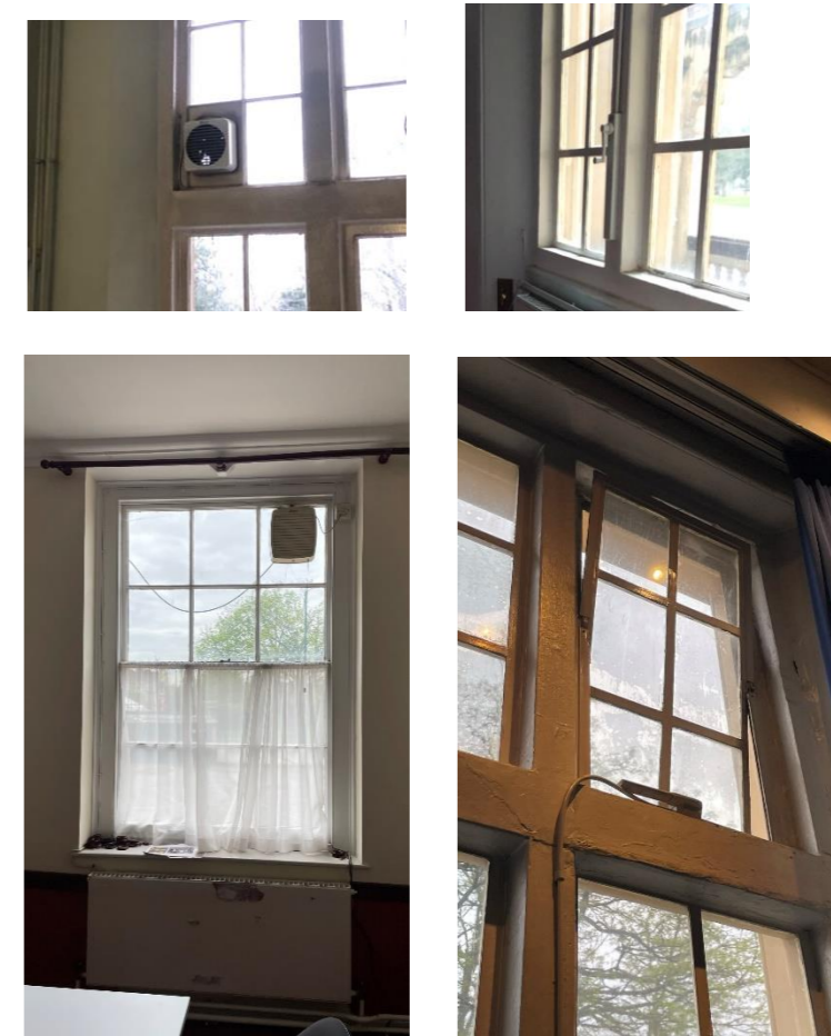
Fig 3. Existing ventilation services and manually openable windows
