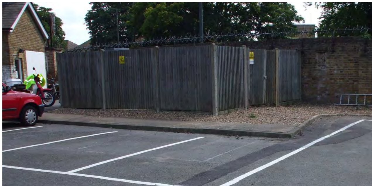
Fig. 2 Existing Location of the Outdoor Transformer
