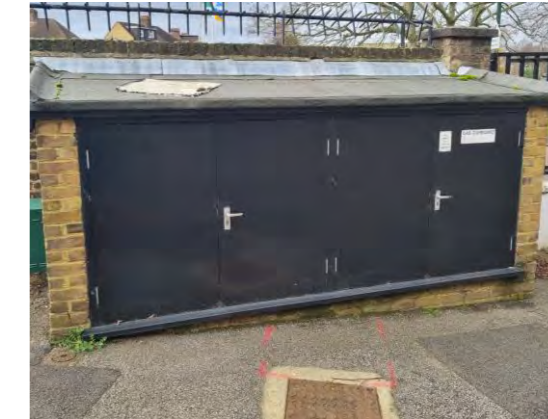
Meter house; Site Boundry
