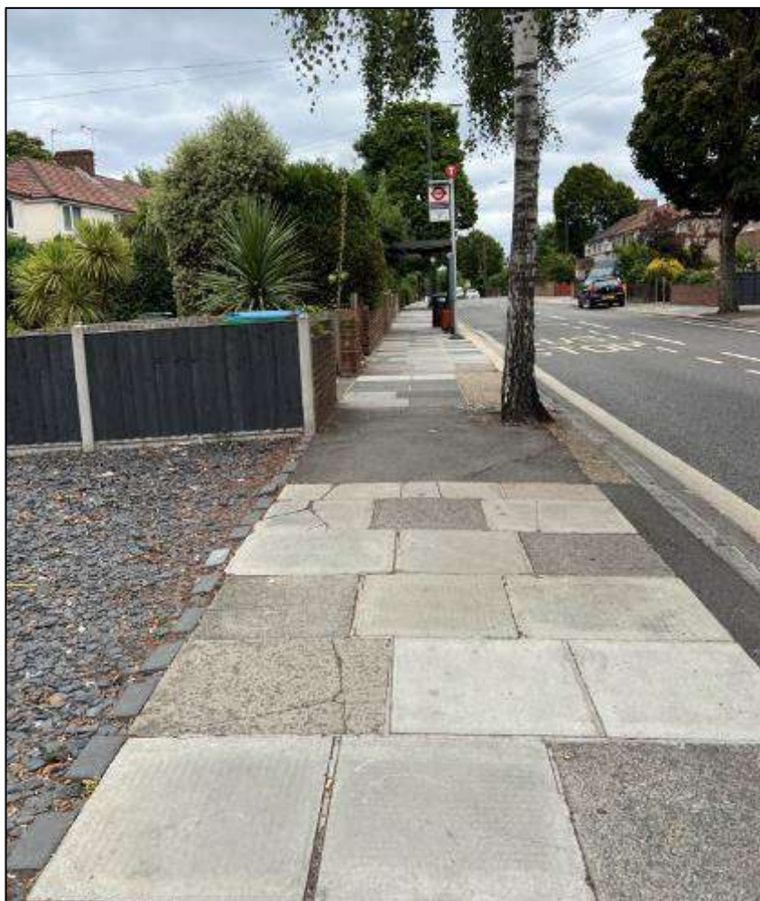
Figure 4.12: Footway on Warren Road
