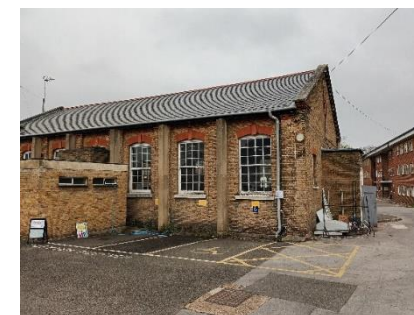
Photo 5 Remedial piers formed of encased steels (back-to-back channels) which anchor remedial ties to the trusses in the Band Practice Hall
