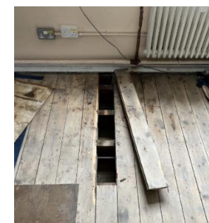
Photo 3 Opening up works showing existing floor joists at the first floor in the Guards House
