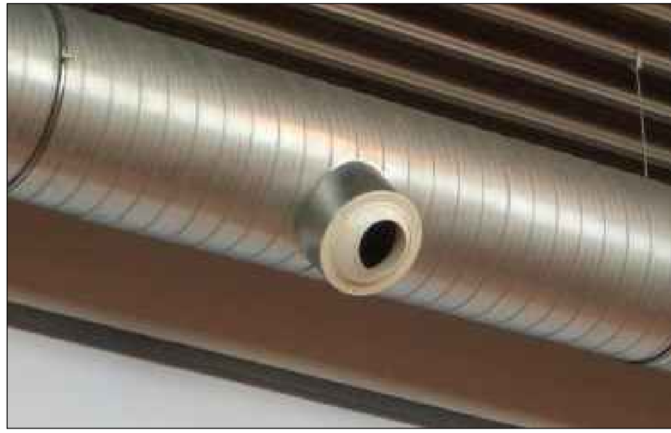
IMAGE 1: WDA LONG THROW NOZZLE FIXED TO SIDE OF CIRCULAR DUCTS
