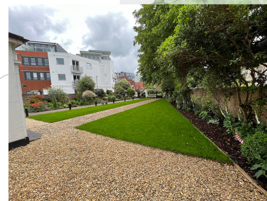
Refurbished Front Garden (works completed)
