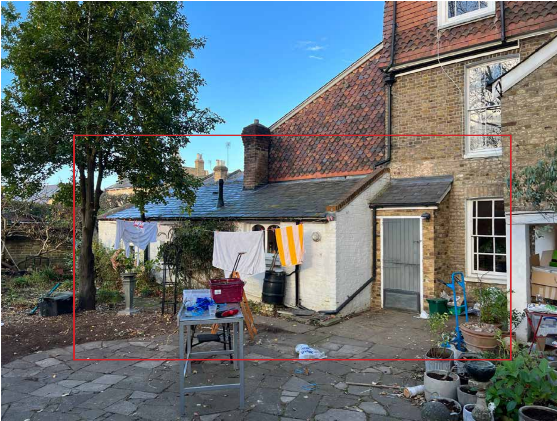
Existing Rear ground floor extension
