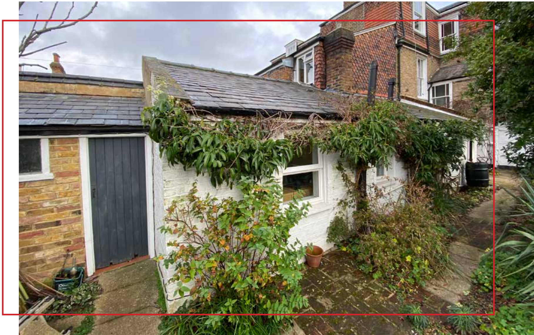
Existing Rear ground floor extension
