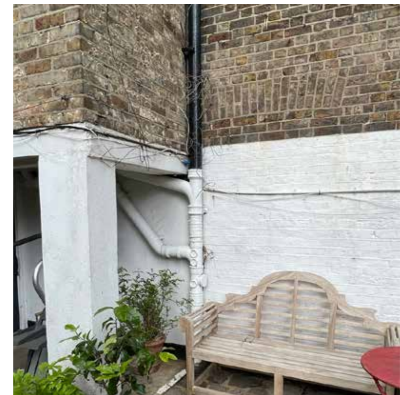
Ground Floor - showing existing brick arch lintel.
