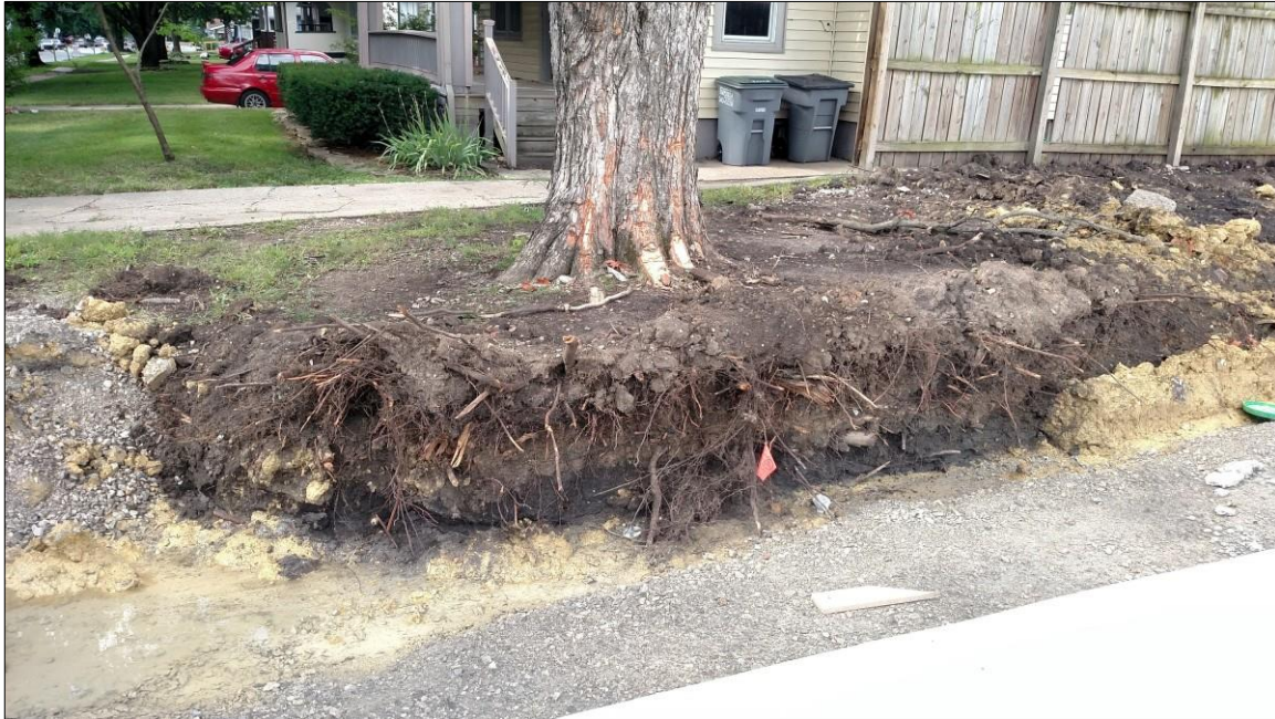
Fig. 1 Damage to roots can both kill and destabilise a tree. Planning work and care can avoid root damage
