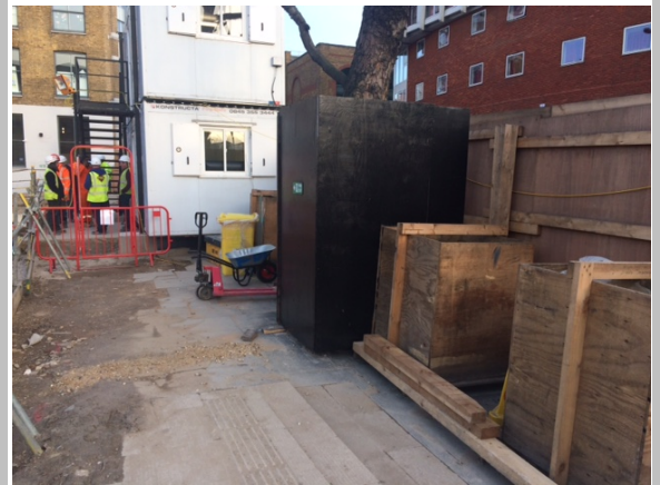
Robust hoarding and temporary concrete ground protection
