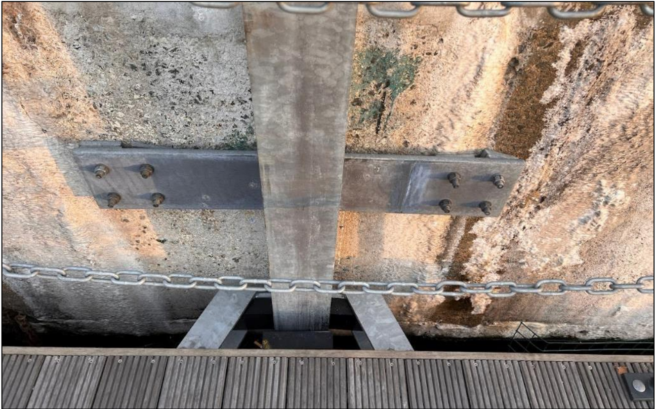
Tide Guide Installation
