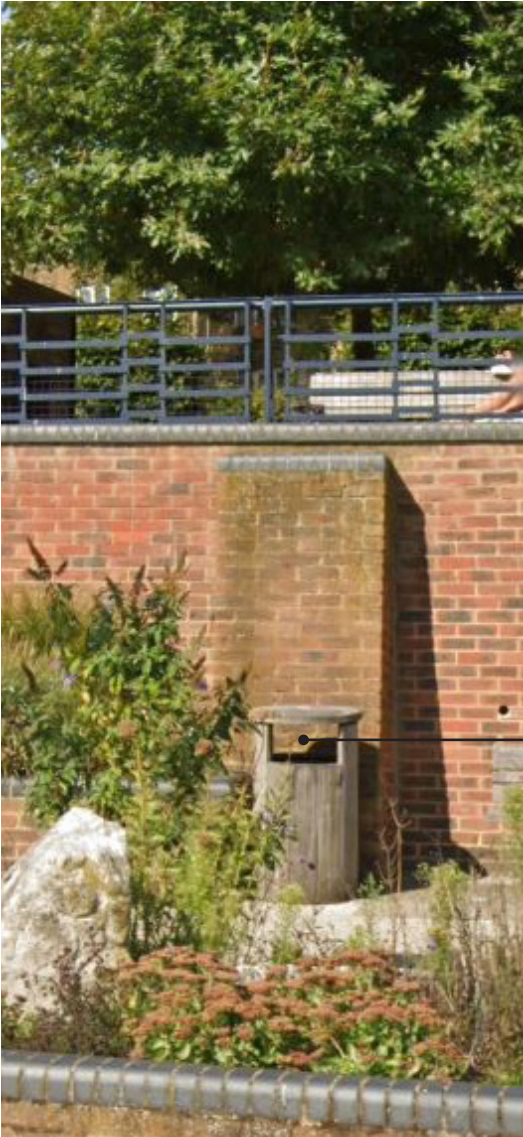
Existing bins to be replaced with same specification
